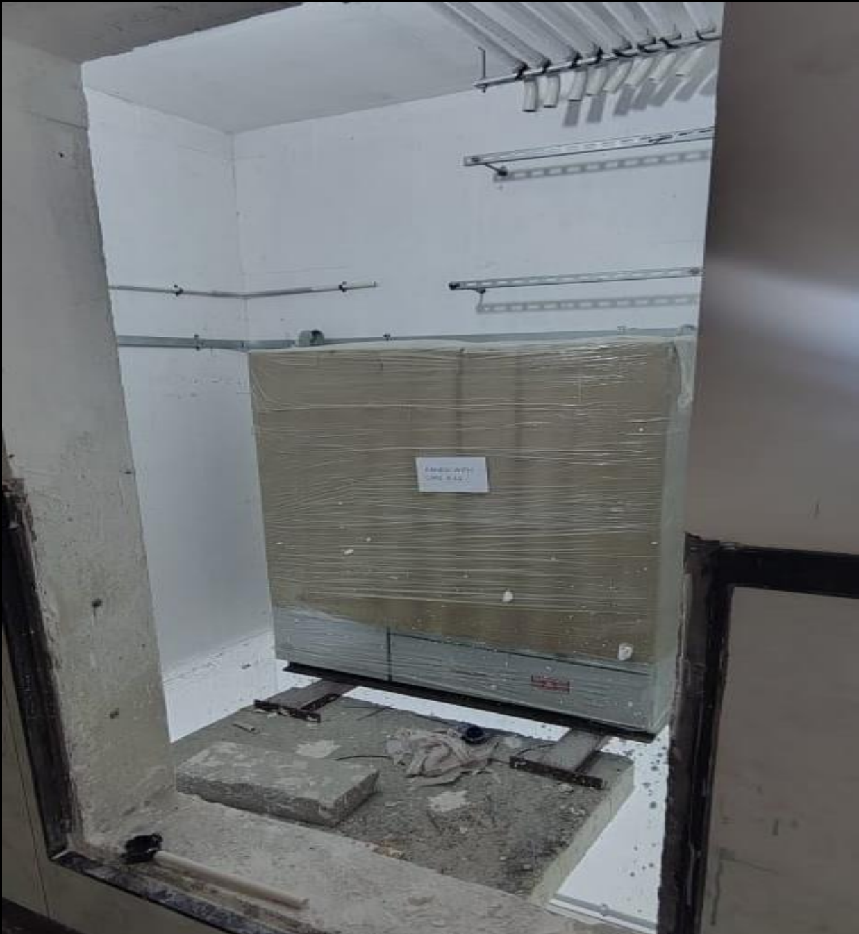
33. Tower A 45 th floor corridor power meter installation done
