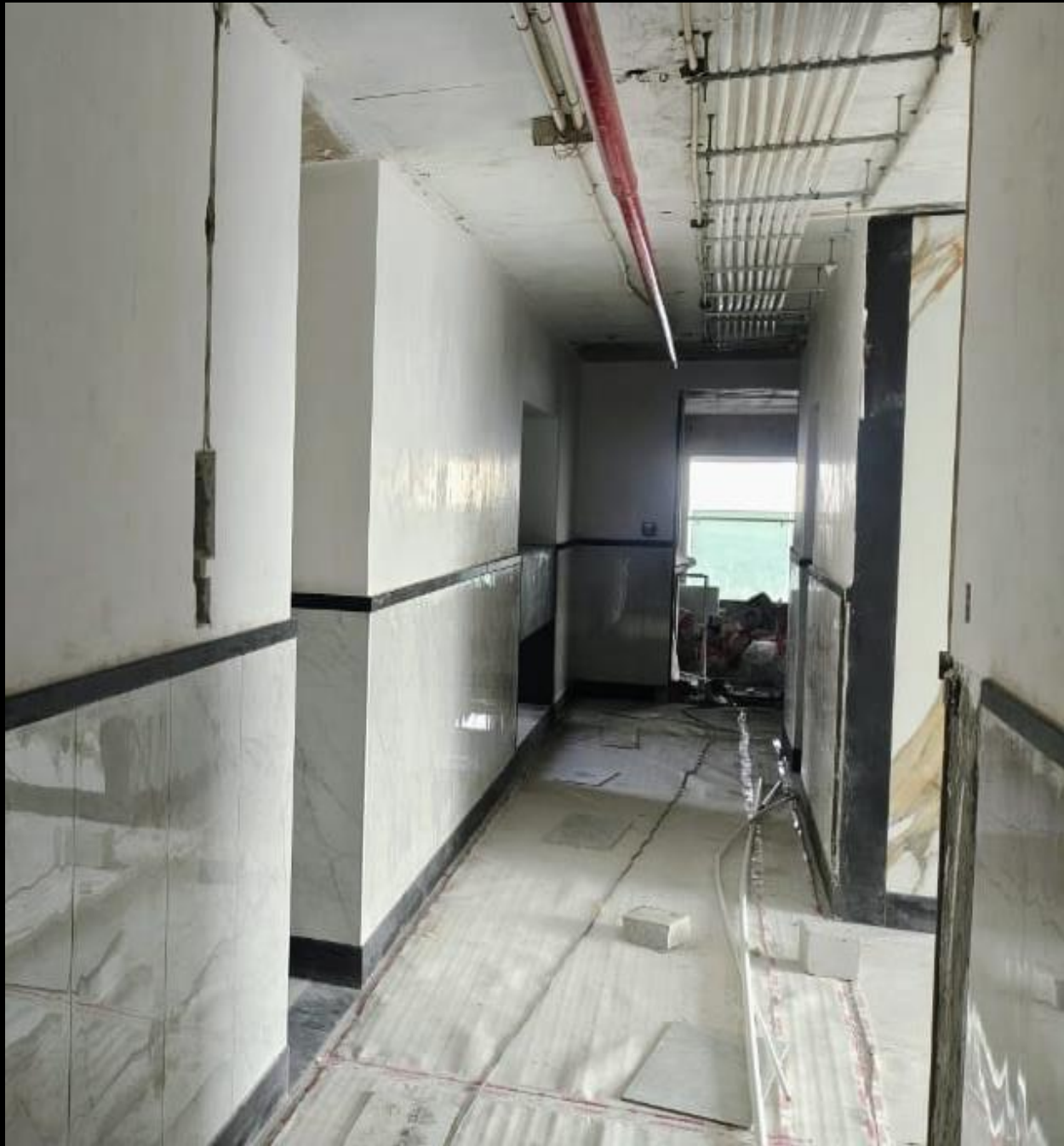
35. Tower B 45 th floor Corridor gypsum paster work in progress
