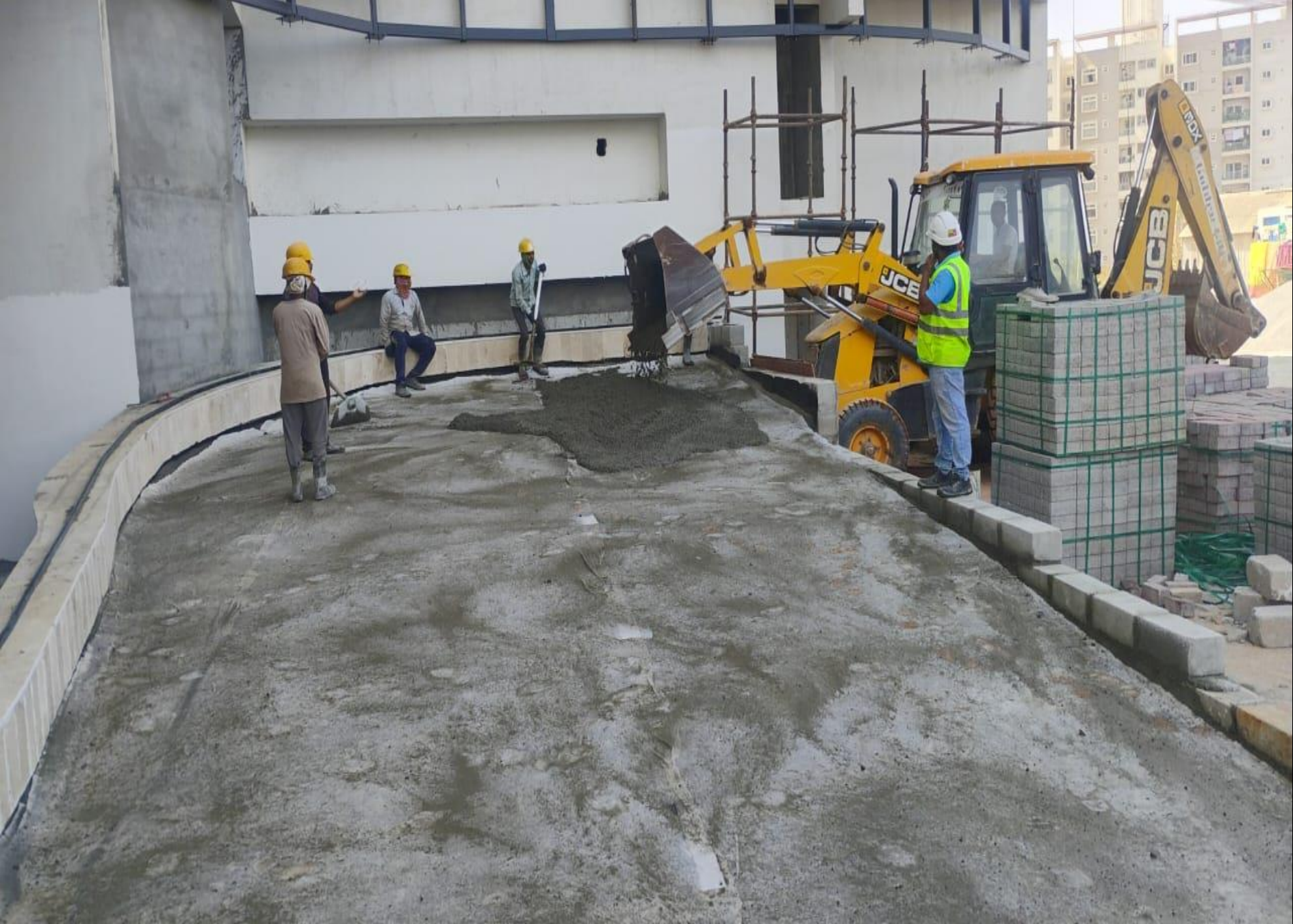
12. Podium ramp north side waterproofing protection screed concrete work in progress
