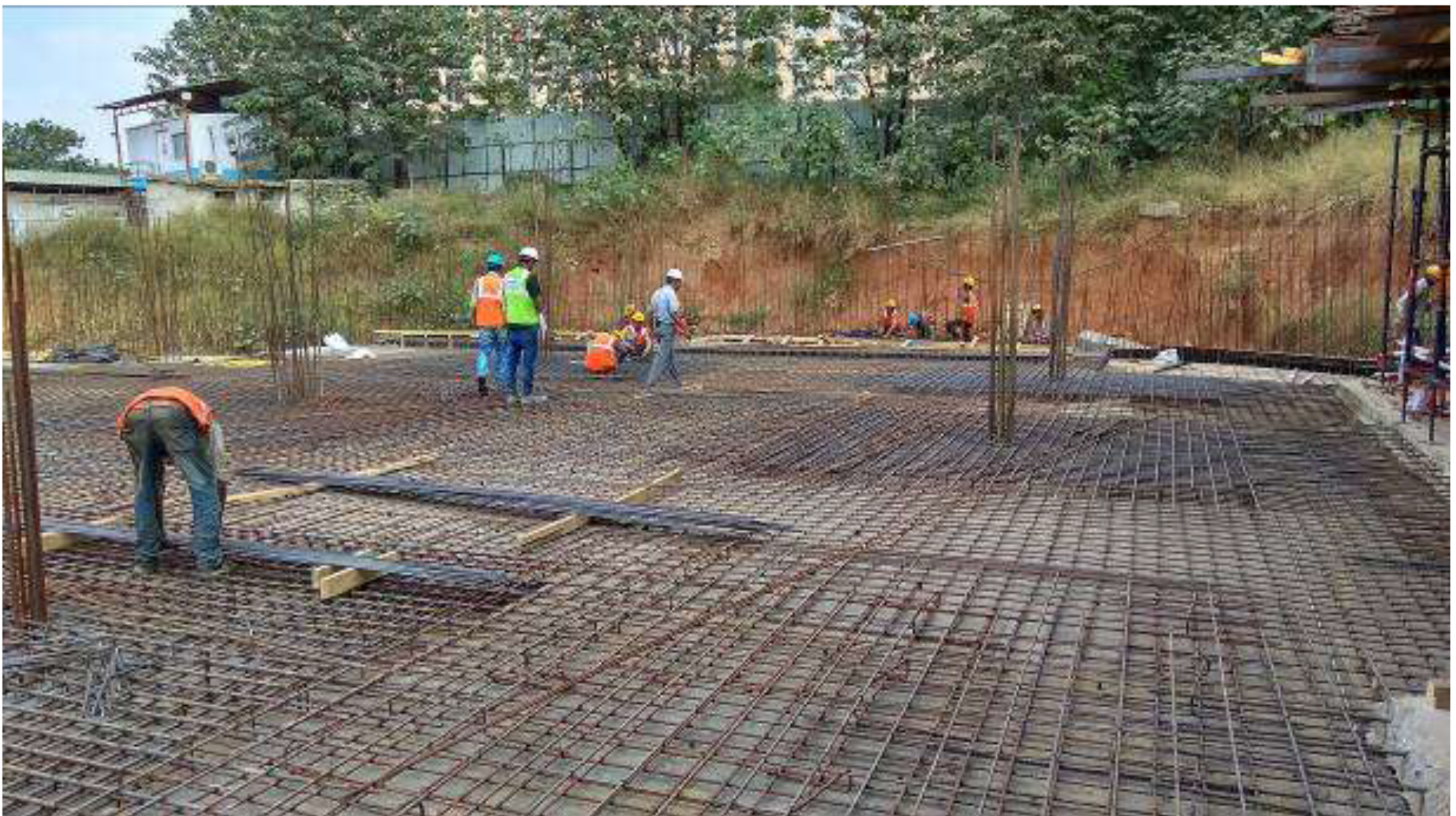
B2 level slab reinforcement work
