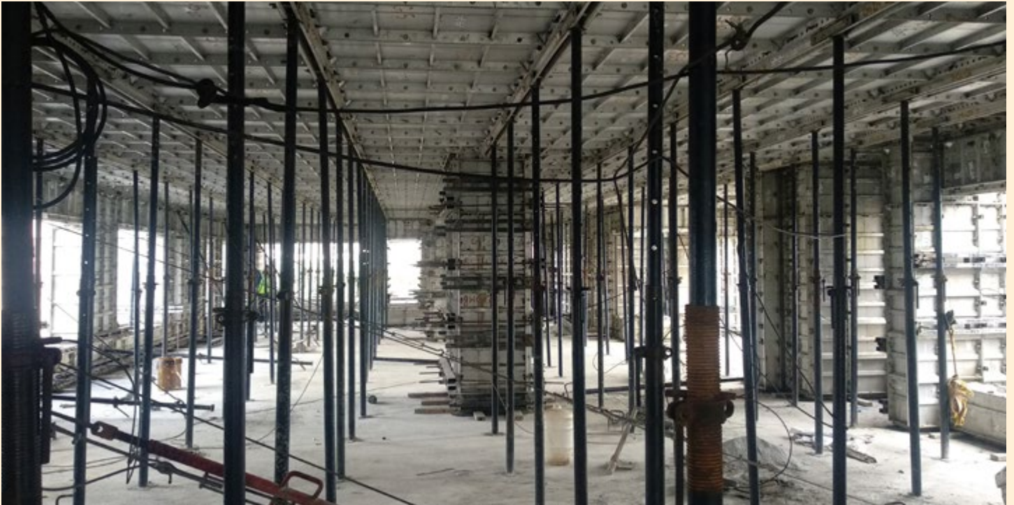
5. Maini after concreting on 3rd Floor
