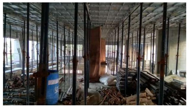
6. De-shuttering of aluminum foam work on 2<sup>nd</sup> Floor
