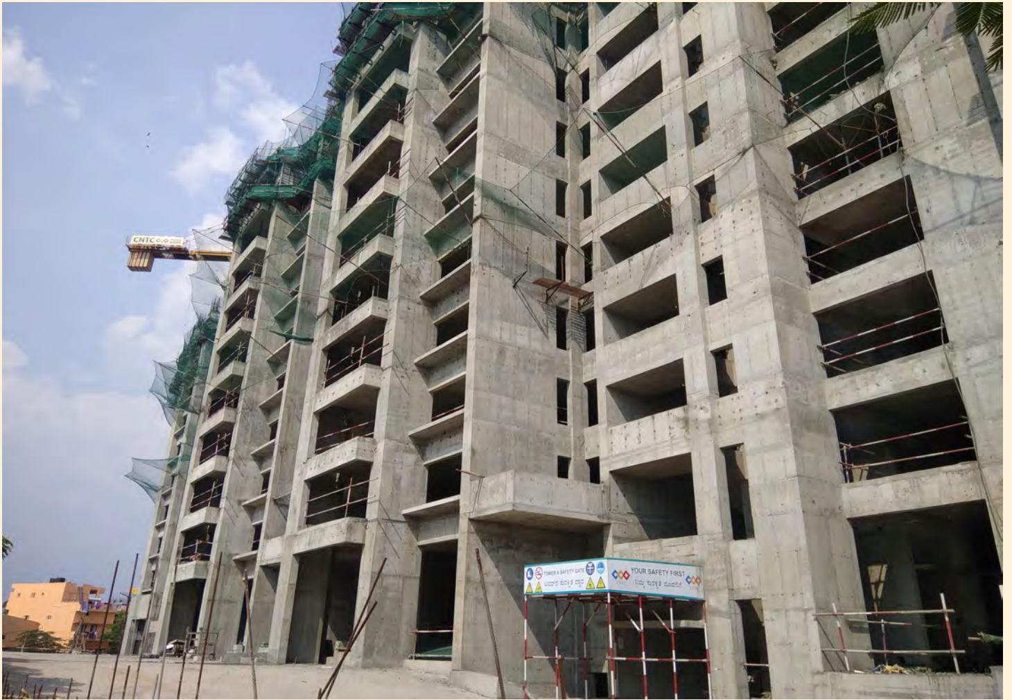
2. Side view with shuttering work in progress
