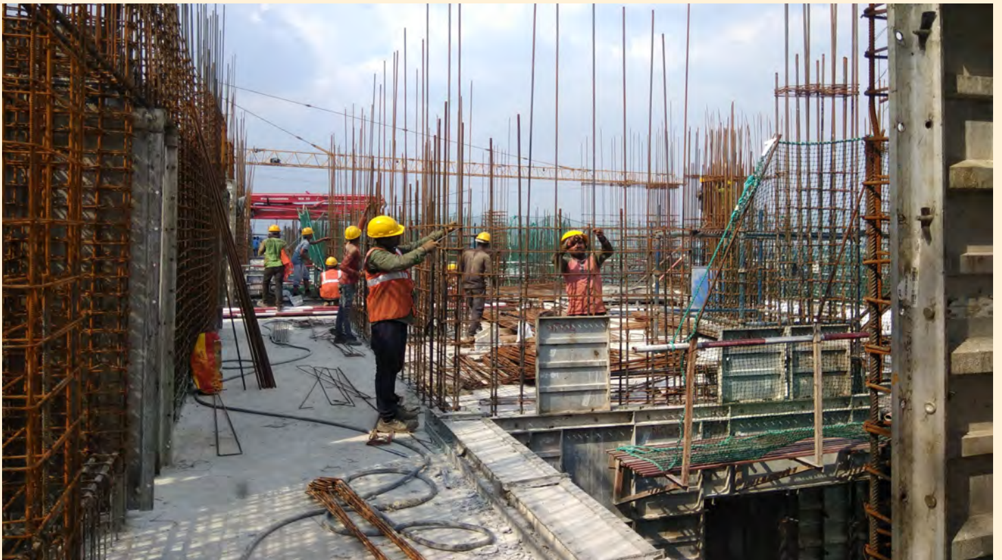
3. Rebar structure on 12th slab
