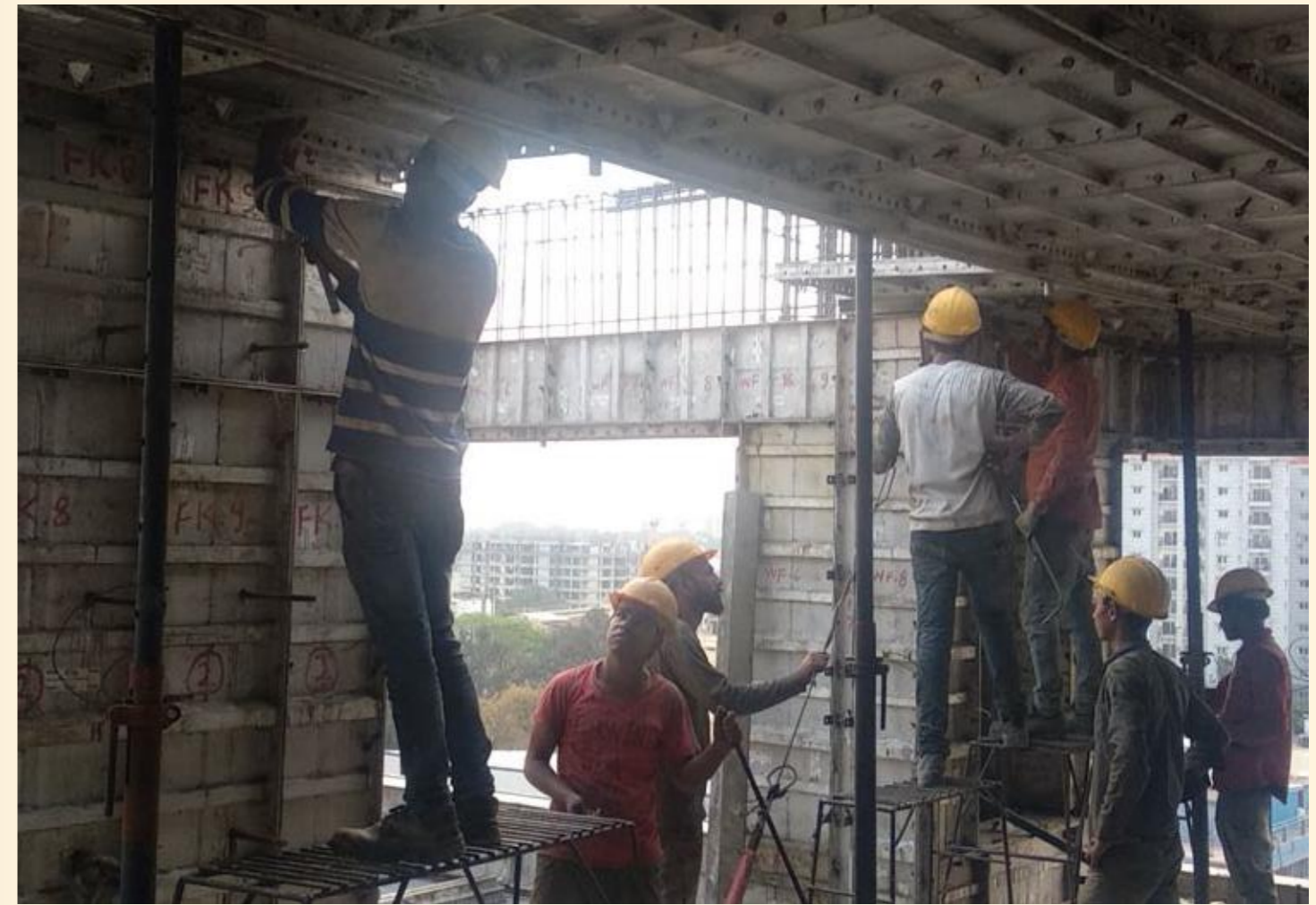
3. Aluminium form work in progress on 10th slab
