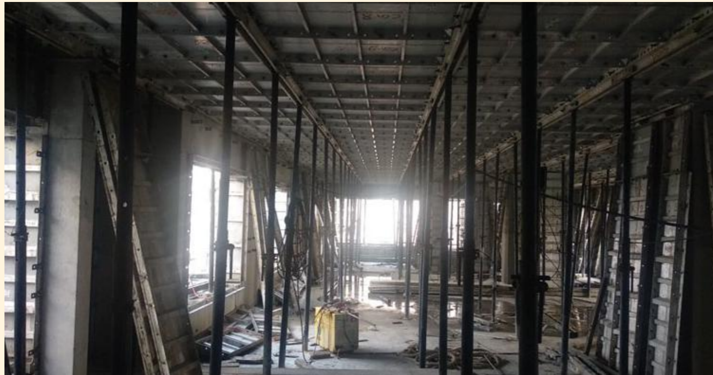
6. Completed Aluminium Form Work on the 9th slab
