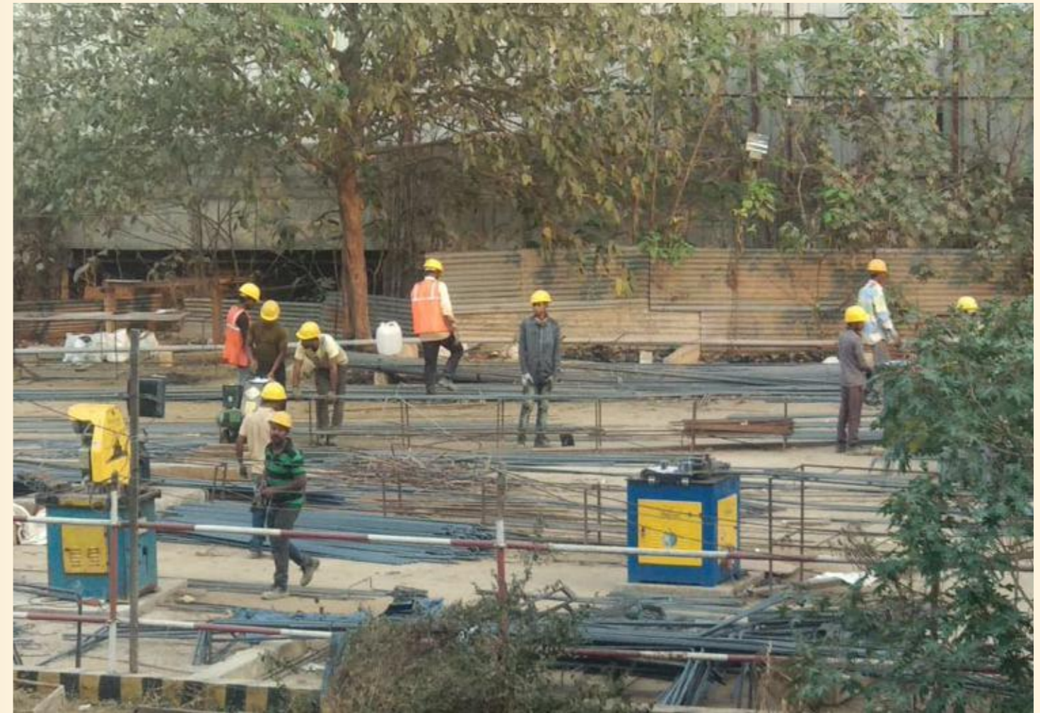
7. Bending, Cutting & Treading of Rebar at Rebar Processing Plant
