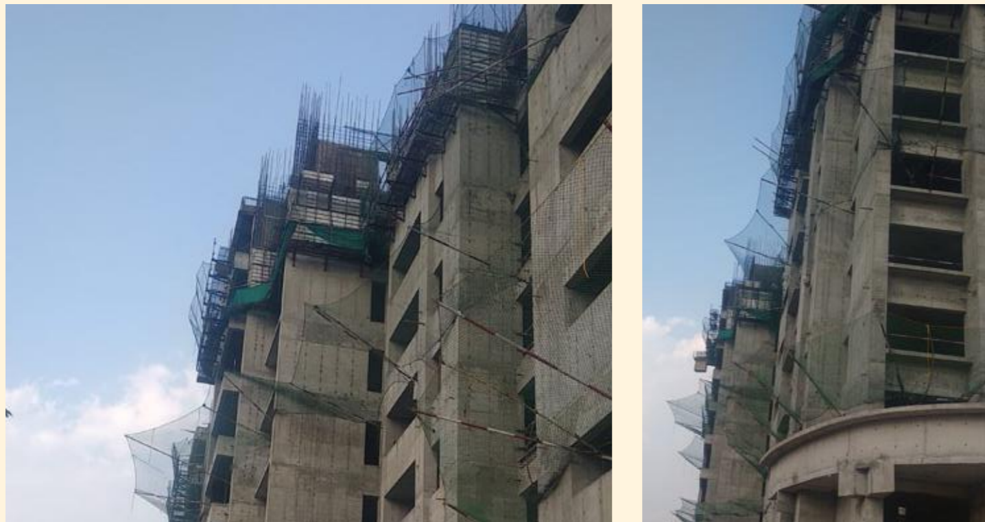
2. Side view of Miani work in progress
