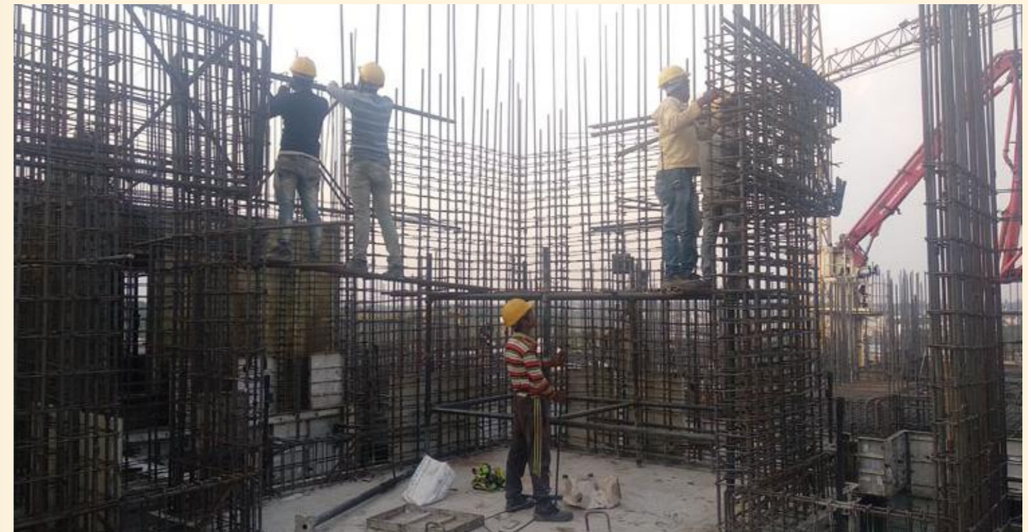
4. Rebar Structure on 10th slab
