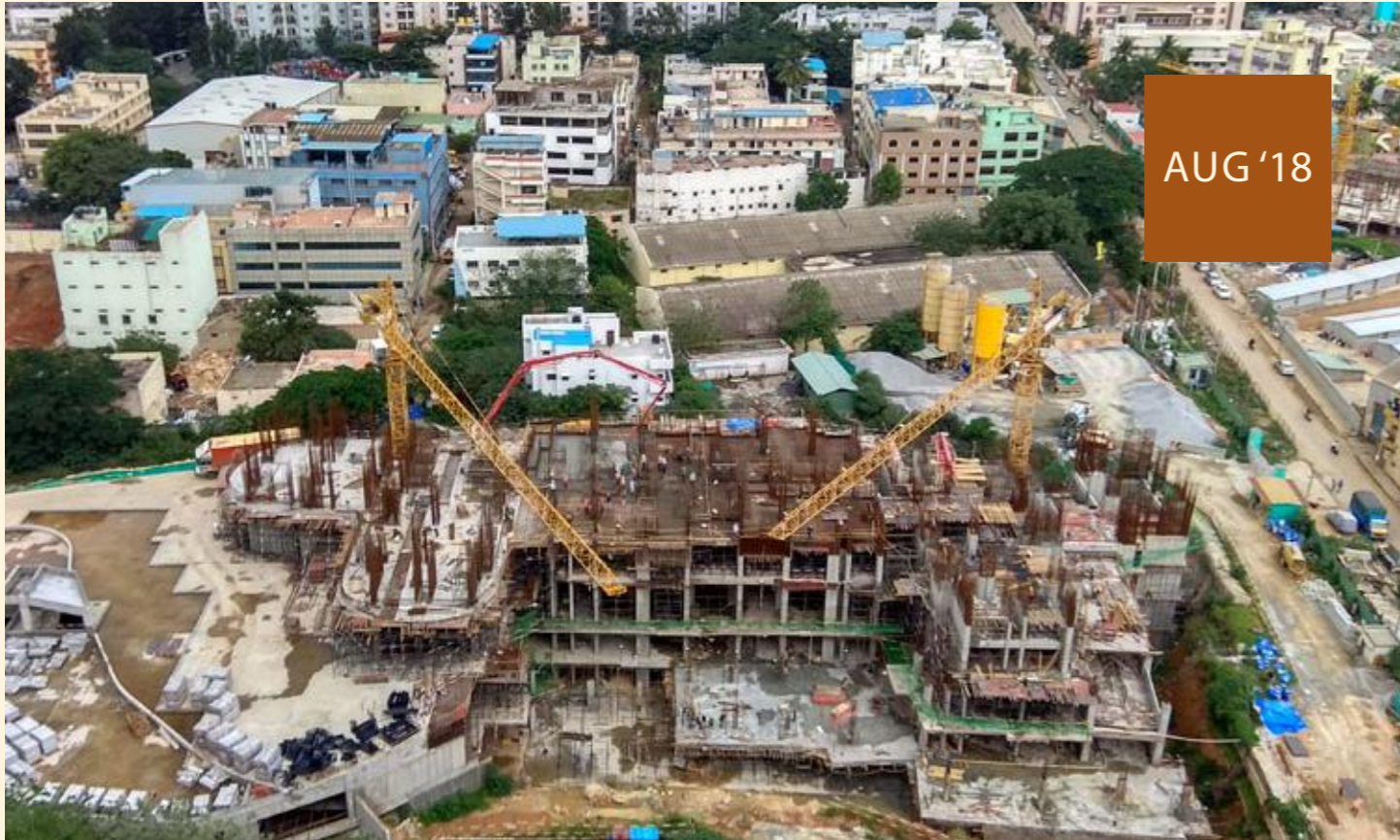
10. Construction progress (Aug '18 - FEB '19)
