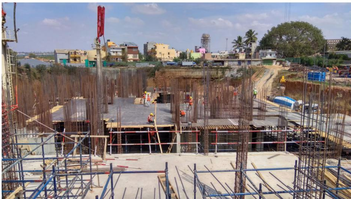
Shear wall reinforcement work from B3 to B2 level
