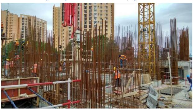
5. Between A-Wing & B Wing column reinforcement work in progress
