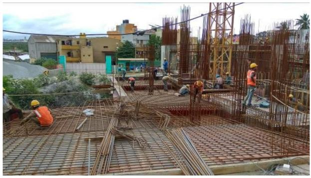
1. Podium Slab Drive way reinforcement work near B-Wing under progress
