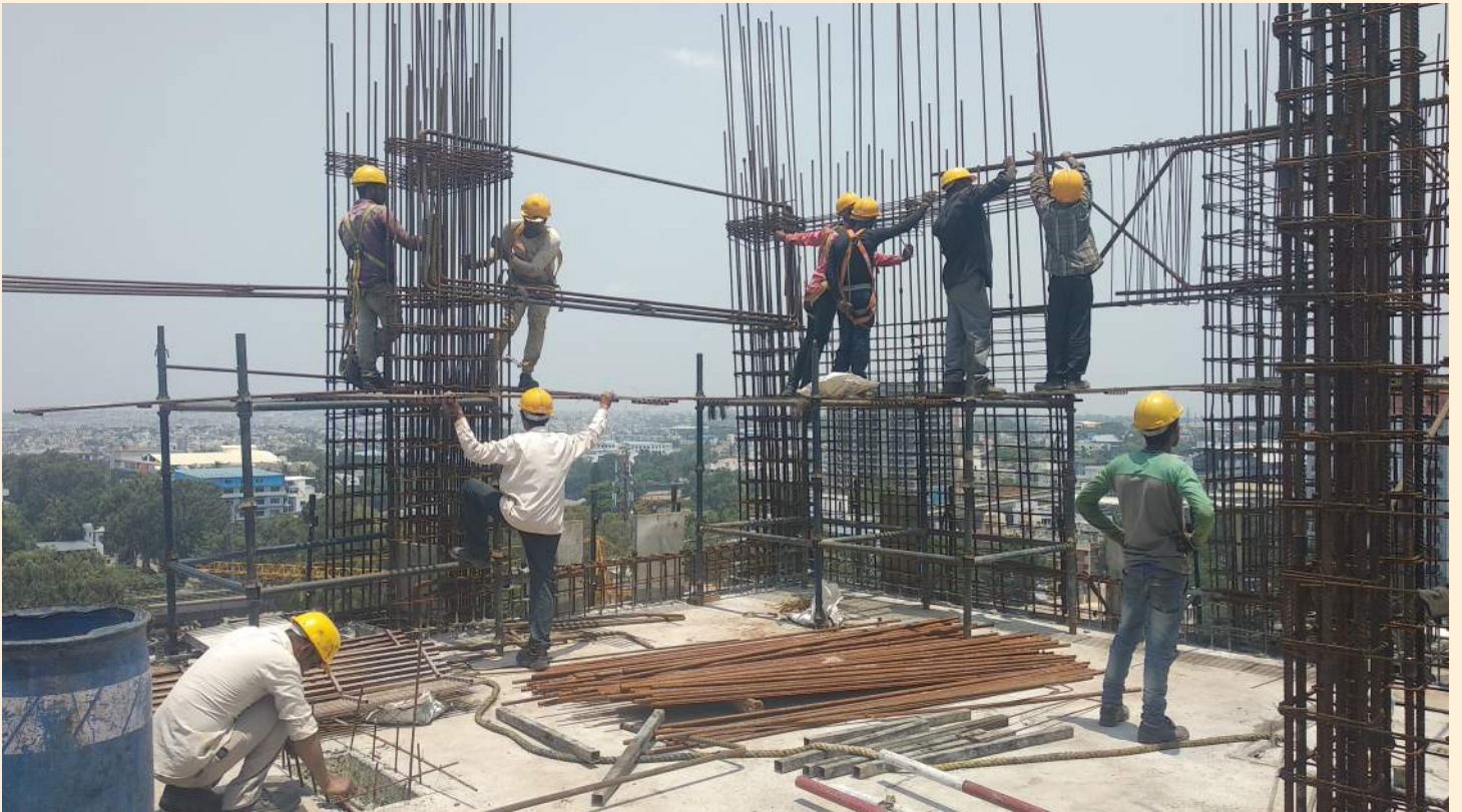
3. Rebar structure of 14th floor work in progress
