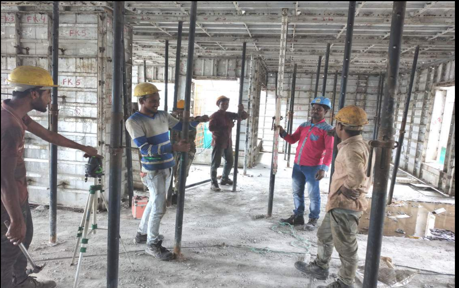
4. Completed Form Work on the 18th floor slab
