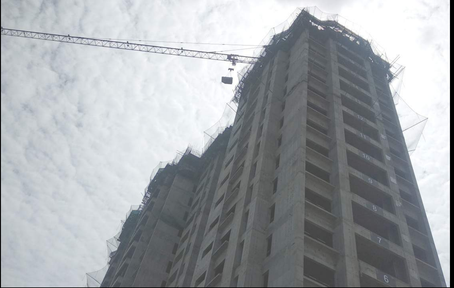
9. Side view with shuttering work in progress
