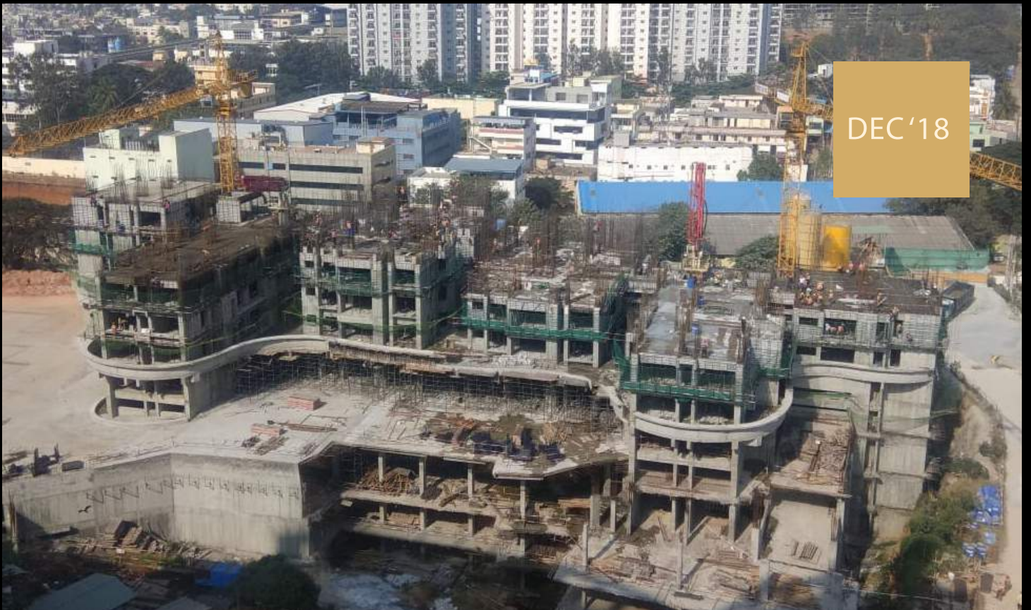
10. Construction progress (DEC '18 - JUNE '19)
