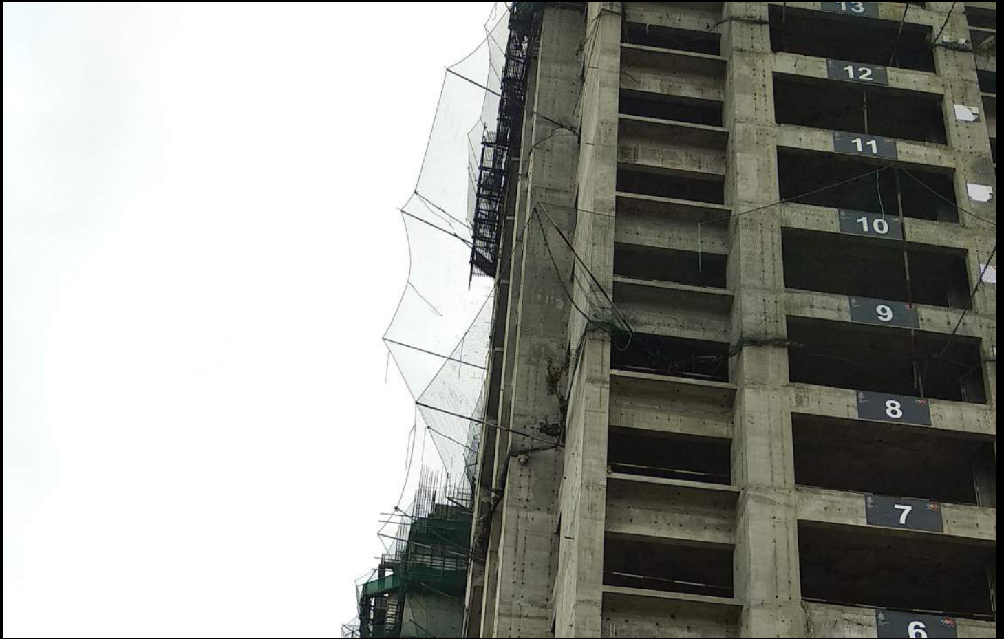
9. Side view with shuttering work in progress
