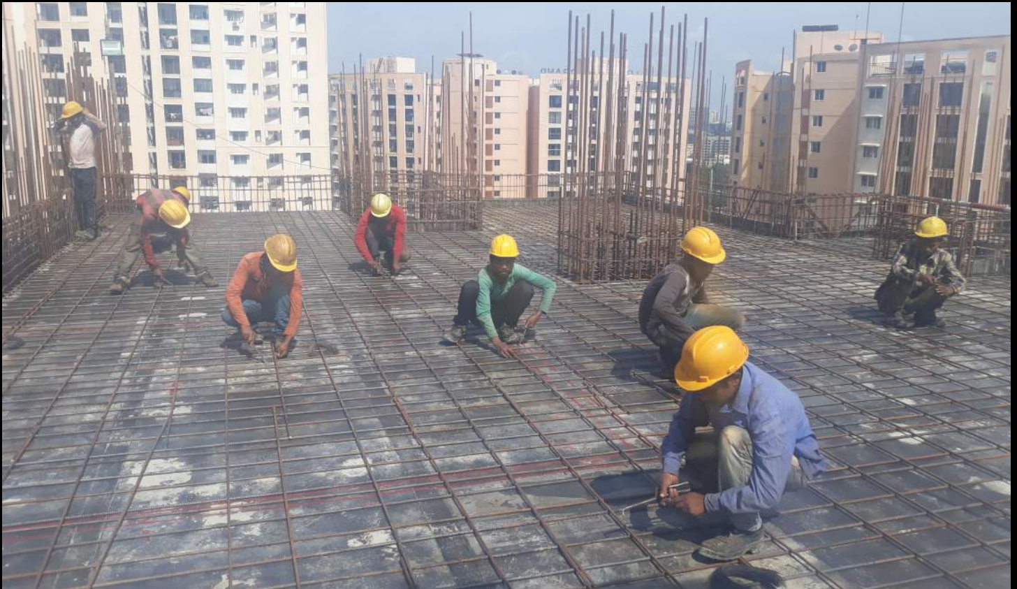
4. Completed Form Work on the 16th floor slab
