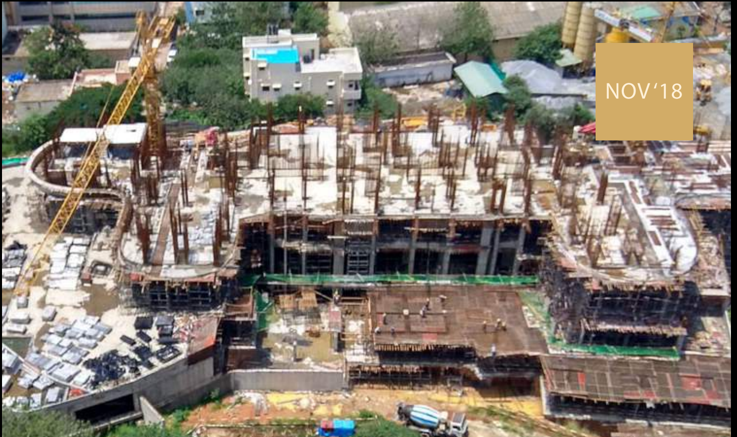
10. Construction progress (NOV '18 - MAY '19)
