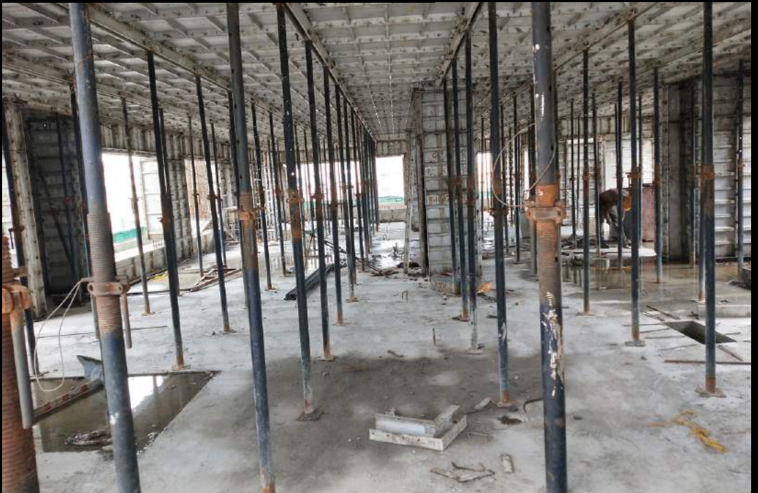
5. Completed Form Work on the 21st floor
