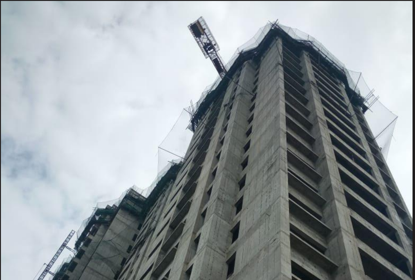
9. Side view with shuttering work in progress
