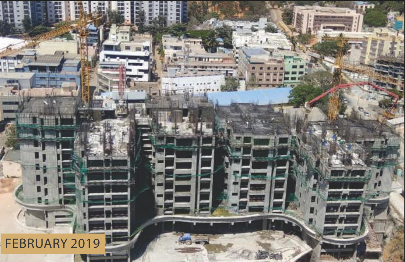
10. Construction progress (FEB'19 - AUG'19)
