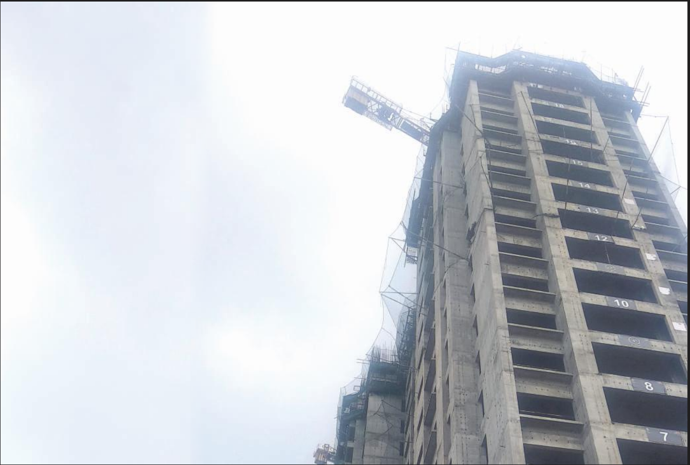
9. Side view with shuttering work in progress
