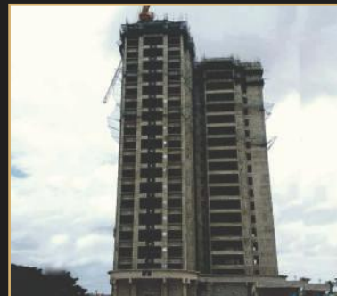
Aug 2019 - 20th floor slab
