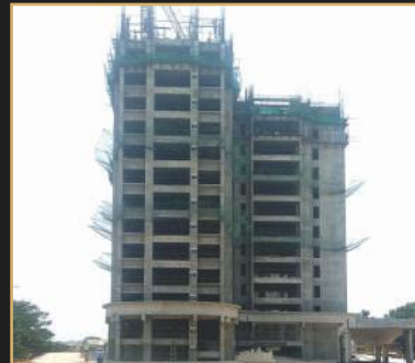
May 2019 - 13th floor slab
