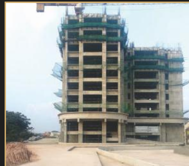
Feb 2019 - 10th floor slab
