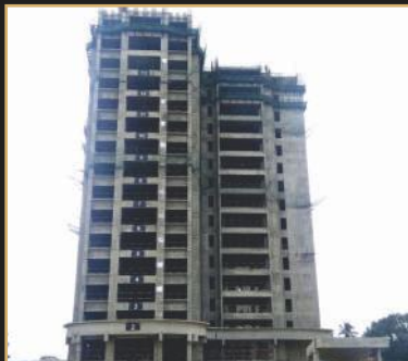
Jun 2019 - 16th floor slab
