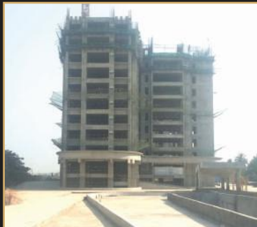
Mar 2019 - 11th floor slab
