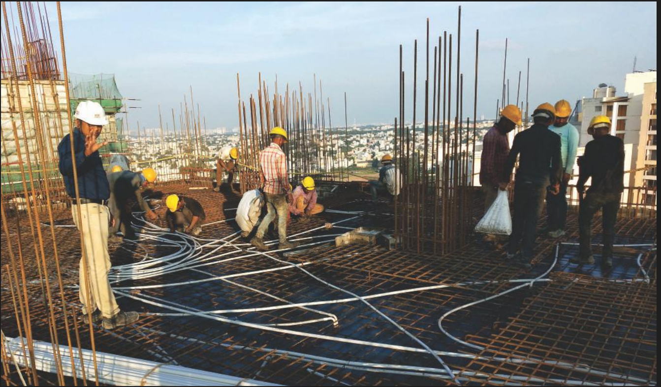
5. Laying of Electrical Conduent on 24th floor
