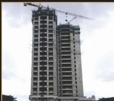
Sep 2019 - 20th floor slab
