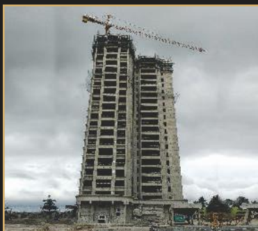
Oct 2019 - 22nd floor slab
