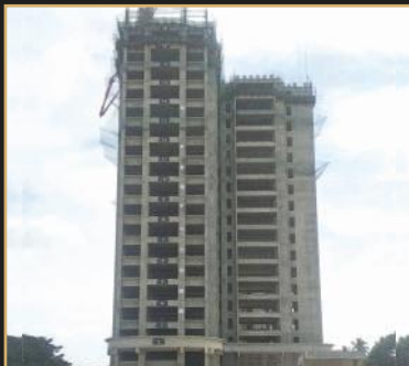
Jul 2019 - 18th floor slab
