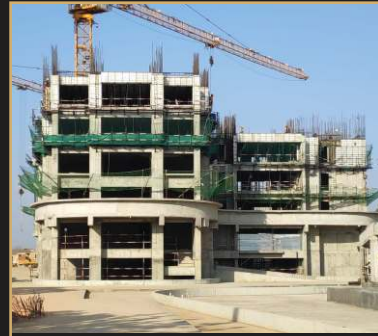
Dec 2018 - 6th floor slab
