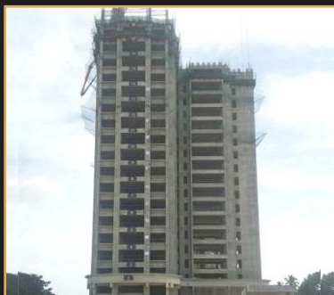
Jul 2019 - 18th floor slab
