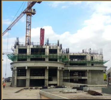
Nov 2018 - 4th floor slab
