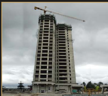
Oct 2019 - 22nd floor slab
