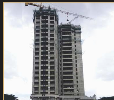
Sep 2019 - 20th floor slab
