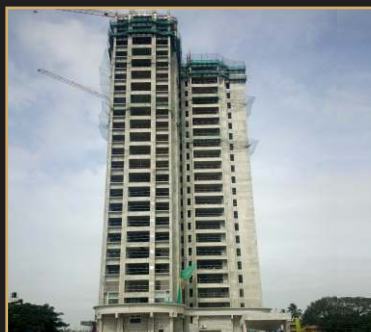
Nov 2019 - 24th floor slab
