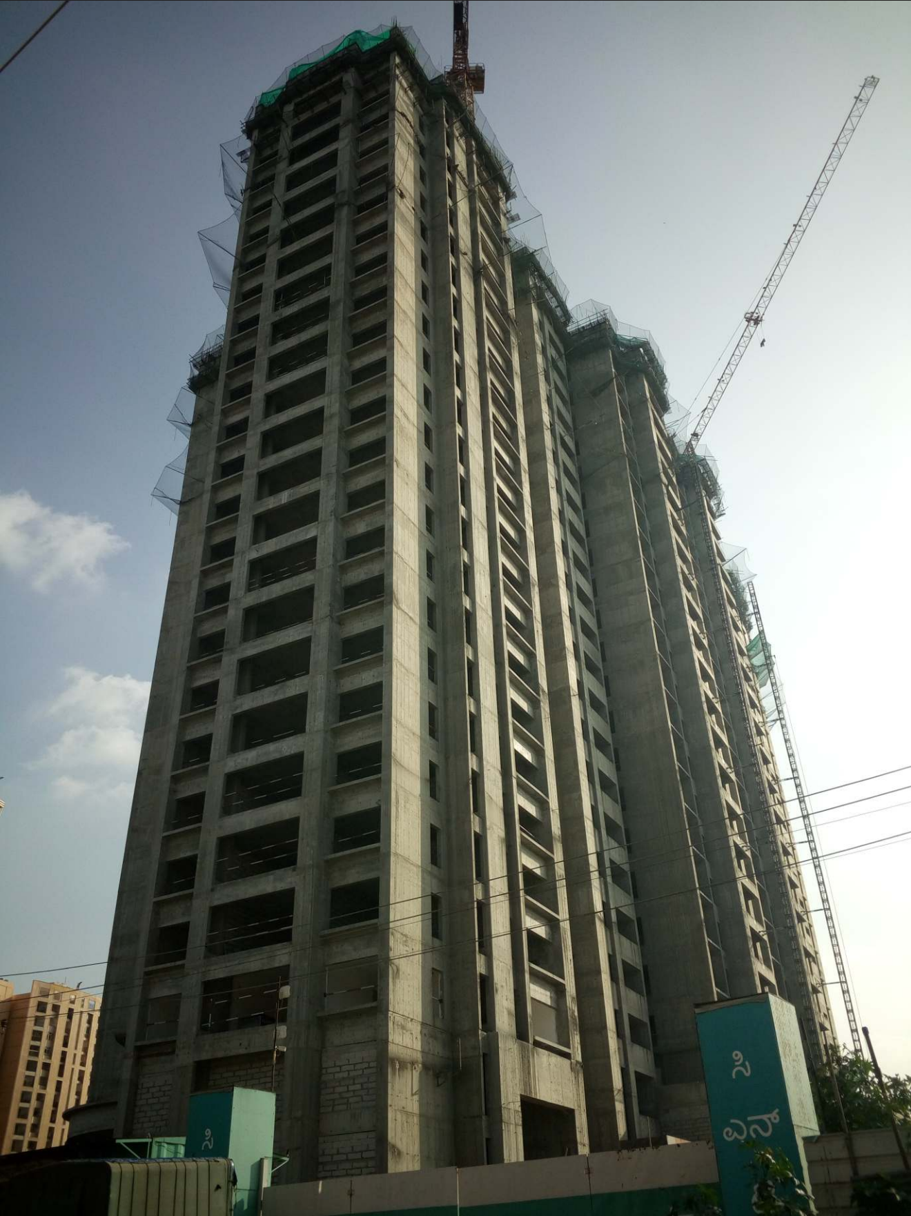
2. View from back gate
