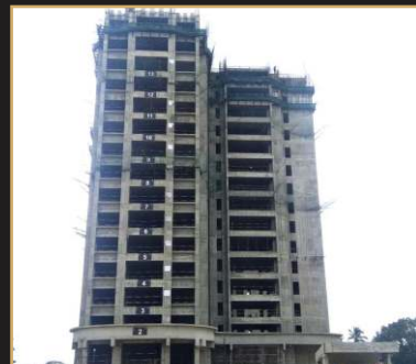
Jun 2019 - 16th floor slab
