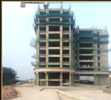
Feb 2019 - 10th floor slab
