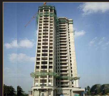
Dec 2019 - 25th floor slab
