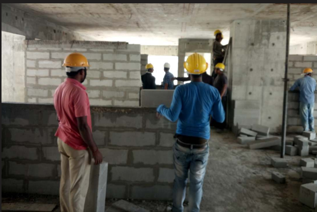
11th floor (Block work WIP)
