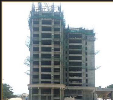
May 2019 - 13th floor slab
