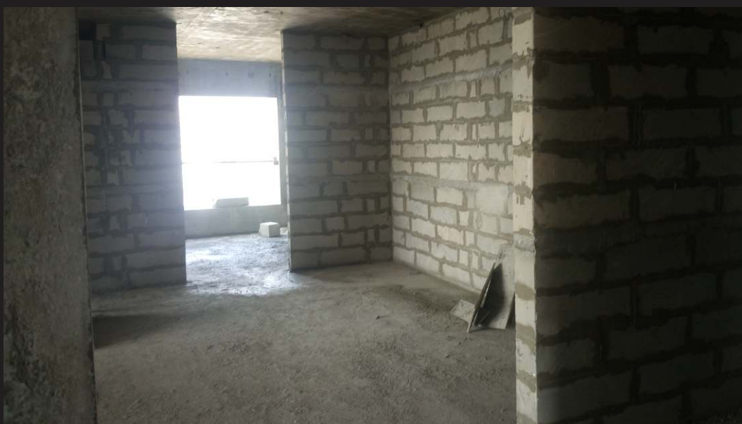
6th to 10th floor (Block work completed)
