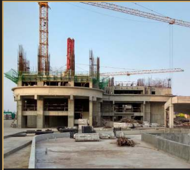
Oct 2018 - 3rd floor slab
