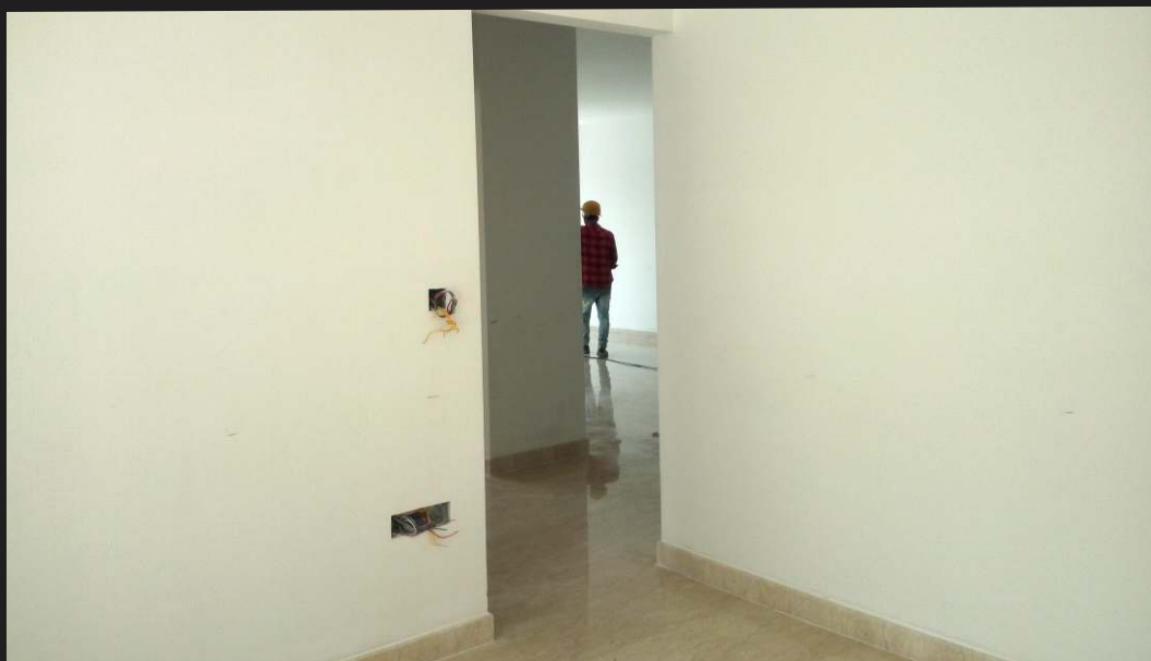
2nd to 5th floor (Plastering work Completed)
