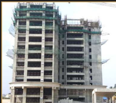
Apr 2019 - 12th floor slab
