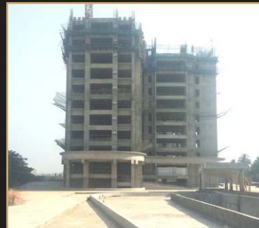
Mar 2019 - 11th floor slab
