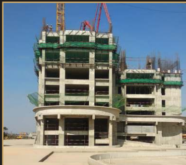
Jan 2019 - 7th floor slab
