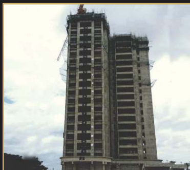
Aug 2019 - 20th floor slab
