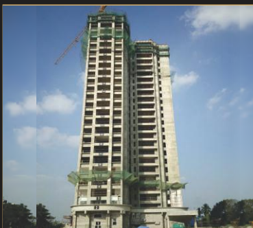
Dec 2019 - 25th floor slab
