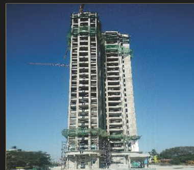
Jan 2020 - 26th floor slab
