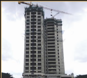
Sep 2019 - 20th floor slab
