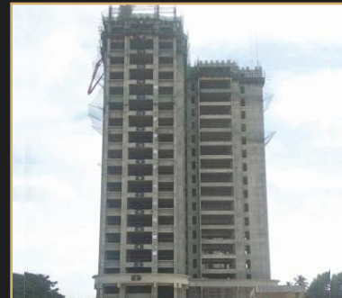
Jul 2019 - 18th floor slab
