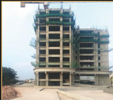
Feb 2019 - 10th floor slab
