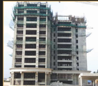
Apr 2019 - 12th floor slab
