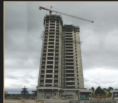
Oct 2019 - 22nd floor slab
