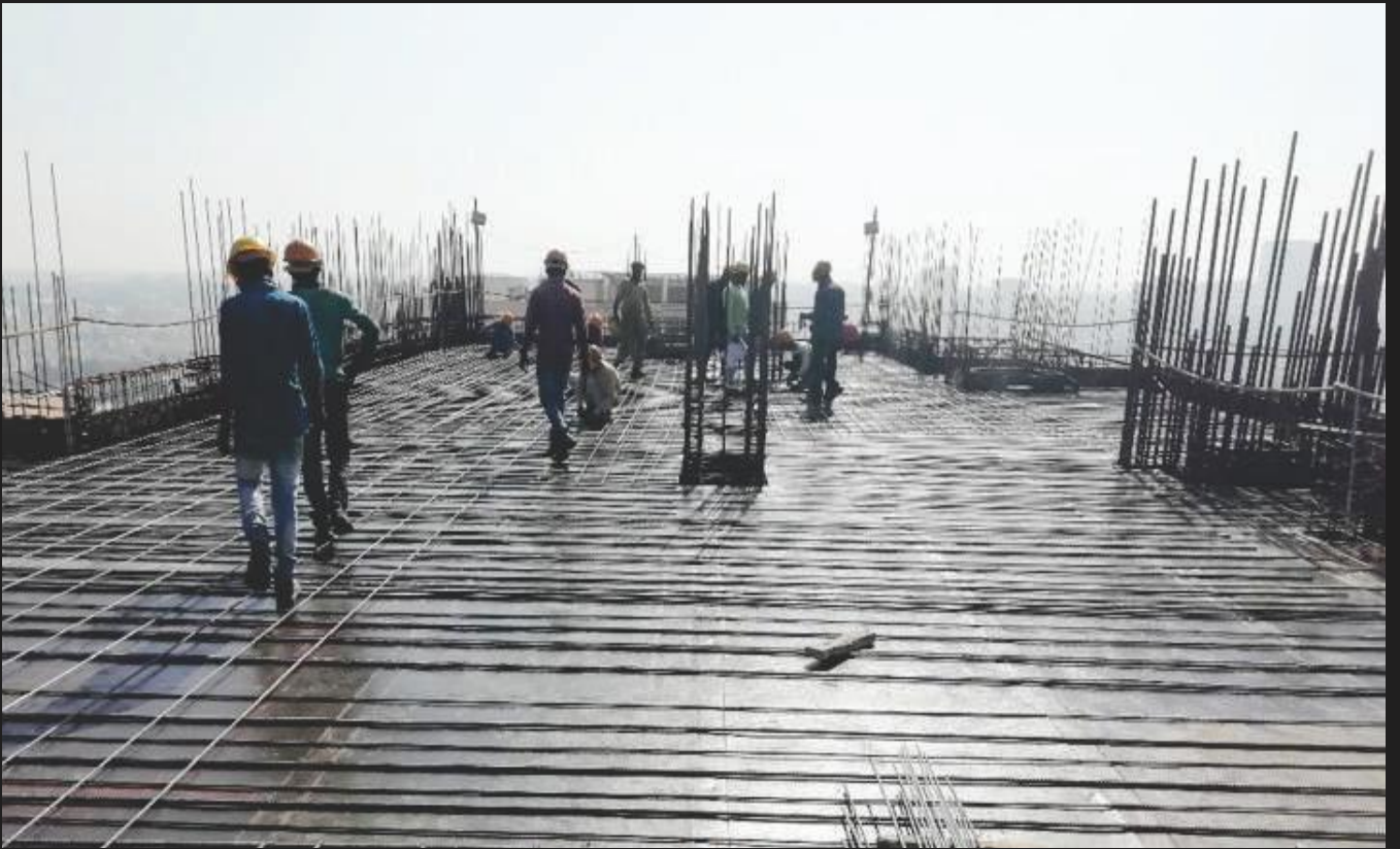
5. Slab reinforcement work in progress on 26th Floor
