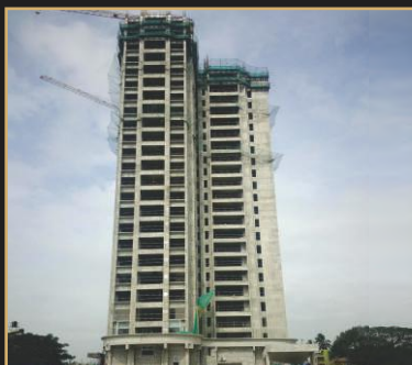
Nov 2019 - 24th floor slab
