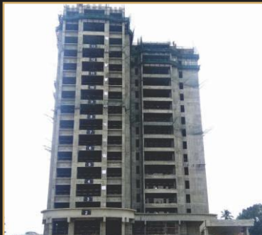
Jun 2019 - 16th floor slab
