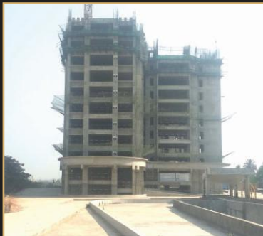
Mar 2019 - 11th floor slab
