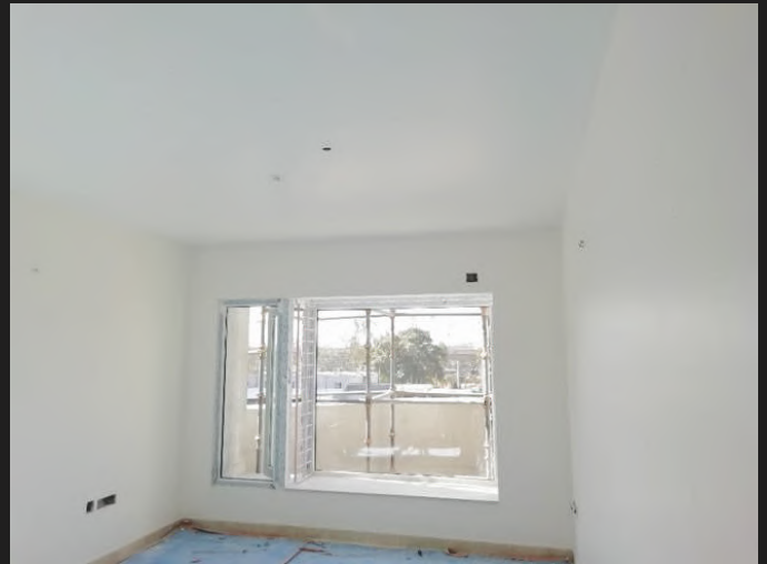
1st coat internal painting work in progress
