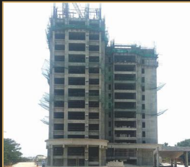
May 2019 - 13th floor slab
