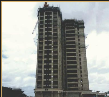
Aug 2019 - 20th floor slab
