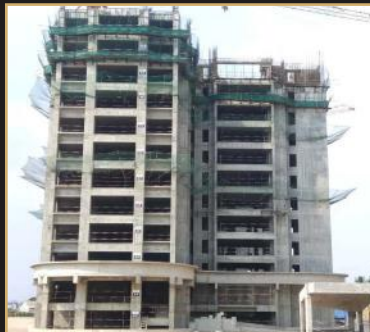
Apr 2019 - 12th floor slab
