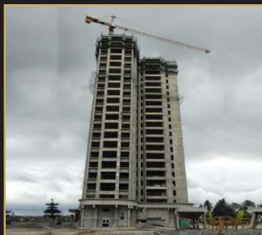
Oct 2019 - 22nd floor slab
