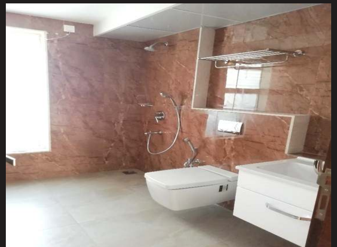
CP & Sanitary fixtures fixing work Completed
