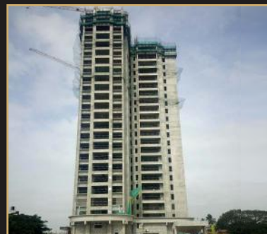
Nov 2019 - 24th floor slab
