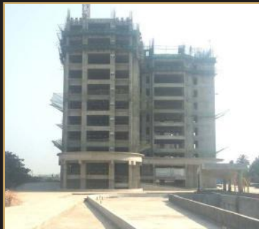
Mar 2019 - 11th floor slab
