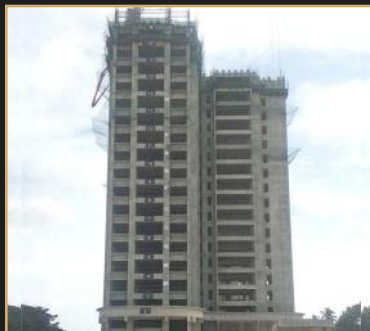
Jul 2019 - 18th floor slab
