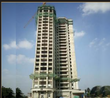
Dec 2019 - 25th floor slab
