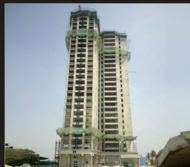
Feb 2020 - 27th floor slab
