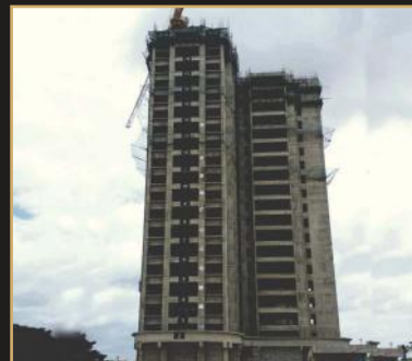
Aug 2019 - 20th floor slab
