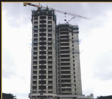
Sep 2019 - 20th floor slab
