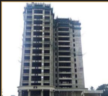
Jun 2019 - 16th floor slab
