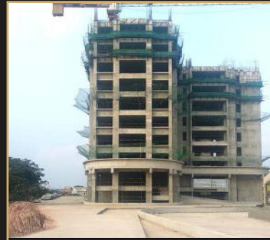
Feb 2019 - 10th floor slab
