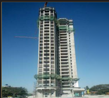
Jan 2020 - 26th floor slab
