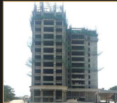
May 2019 - 13th floor slab
