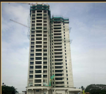
Nov 2019 - 24th floor slab
