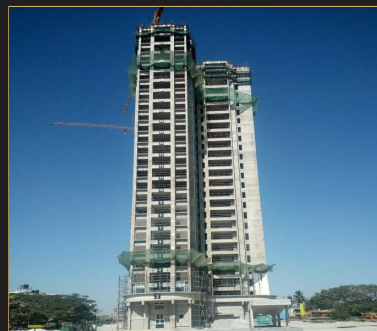
Jan 2020 - 26th floor slab
