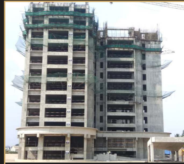
Apr 2019 - 12th floor slab
