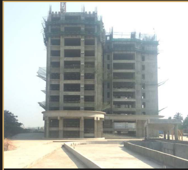
Mar 2019 - 11th floor slab
