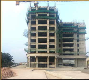
Feb 2019 - 10th floor slab
