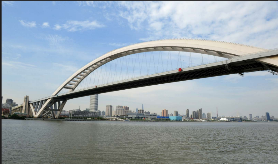
Shanghai Lupu Bridge
