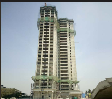
Feb 2020 - 27th floor slab
