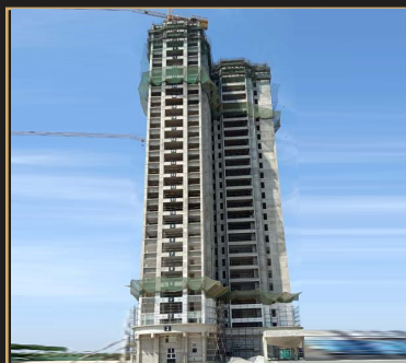
Mar 2020 - 28th floor slab
