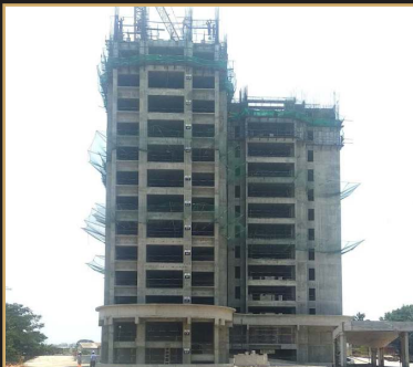
May 2019 - 13th floor slab
