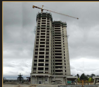
Oct 2019 - 22nd floor slab
