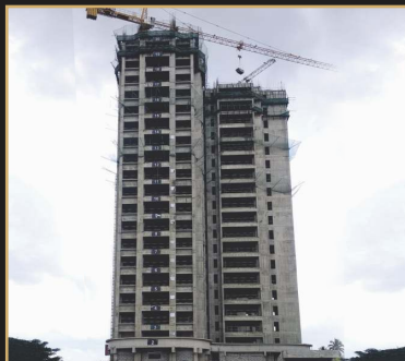
Sep 2019 - 20th floor slab
