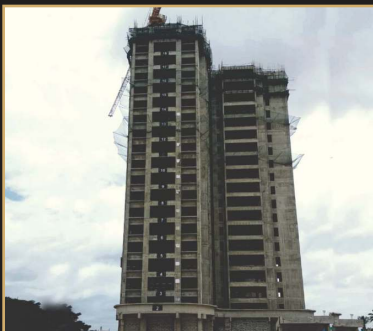
Aug 2019 - 20th floor slab
