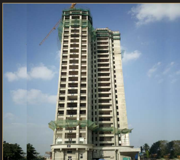
Dec 2019 - 25th floor slab
