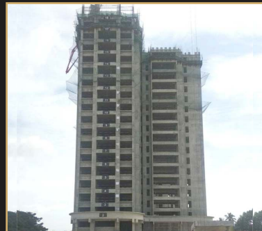
Jul 2019 - 18th floor slab
