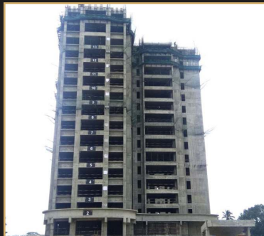
Jun 2019 - 16th floor slab
