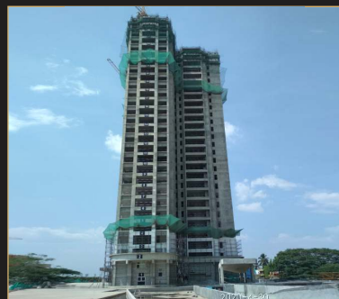
Apr 2020 - 28th floor slab
