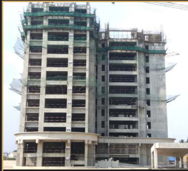
Apr 2019 - 12th floor slab
