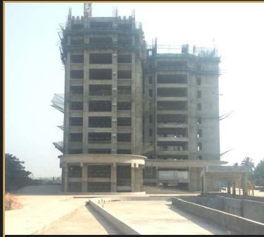
Mar 2019 - 11th floor slab
