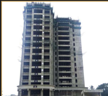
Jun 2019 - 16th floor slab
