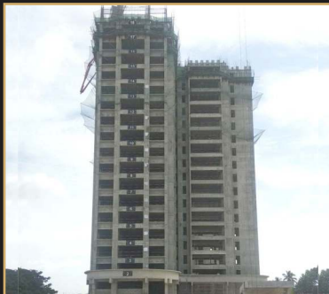
Jul 2019 - 18th floor slab
