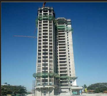
Jan 2020 - 26th floor slab
