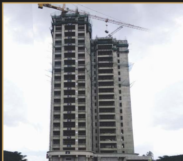
Sep 2019 - 20th floor slab
