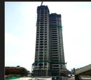
May 2020 - 29th floor slab
