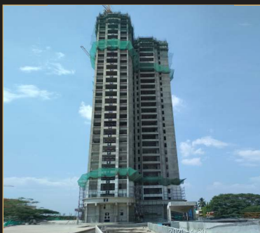
Apr 2020 - 28th floor slab
