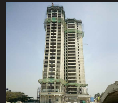
Feb 2020 - 27th floor slab
