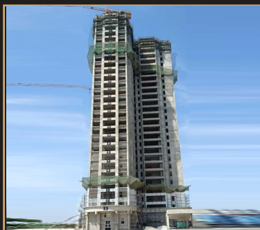
Mar 2020 - 28th floor slab
