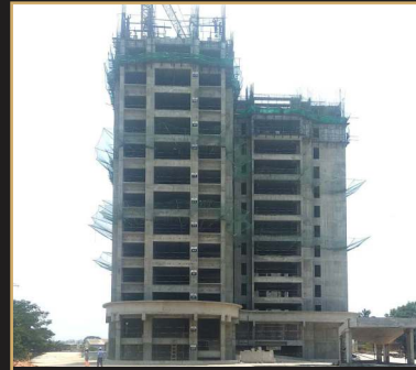
May 2019 - 13th floor slab
