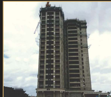
Aug 2019 - 20th floor slab
