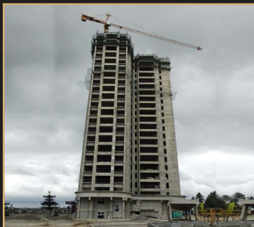
Oct 2019 - 22nd floor slab
