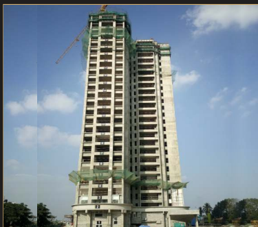
Dec 2019 - 25th floor slab
