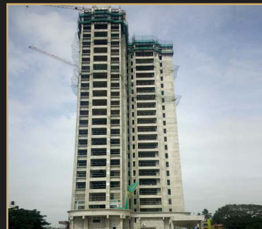
Nov 2019 - 24th floor slab
