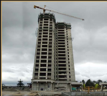
Oct 2019 - 22nd floor slab
