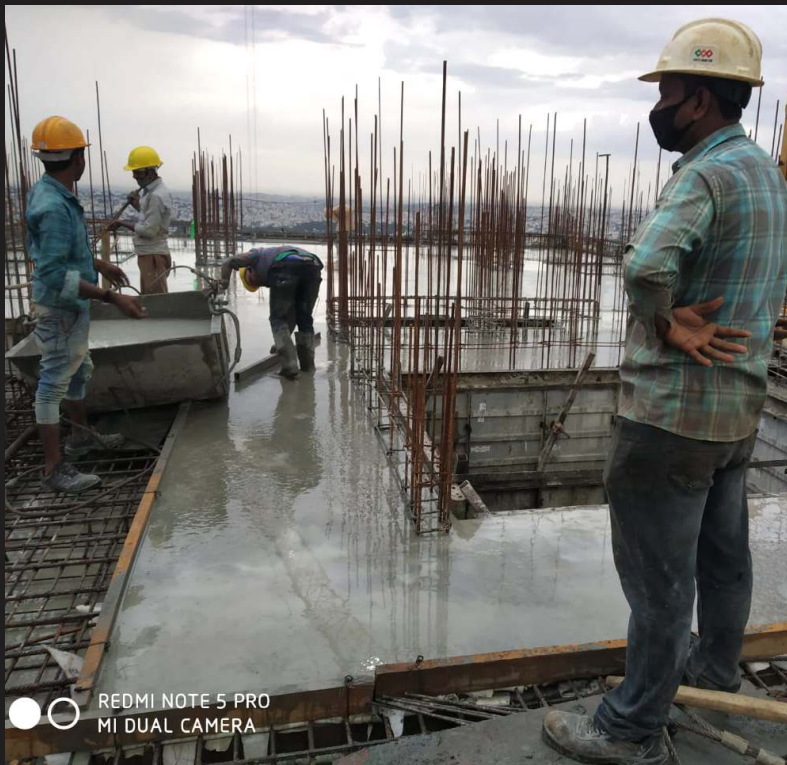
6. Concrete pouring on 30 th floor
