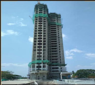
Apr 2020 - 28th floor slab
