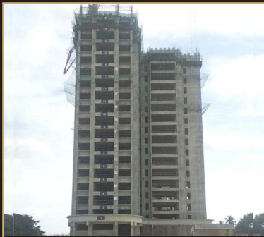
Jul 2019 - 18th floor slab
