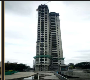
Jun 2020 - 30th floor slab
