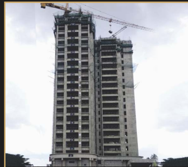
Sep 2019 - 20th floor slab
