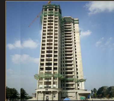
Dec 2019 - 25th floor slab
