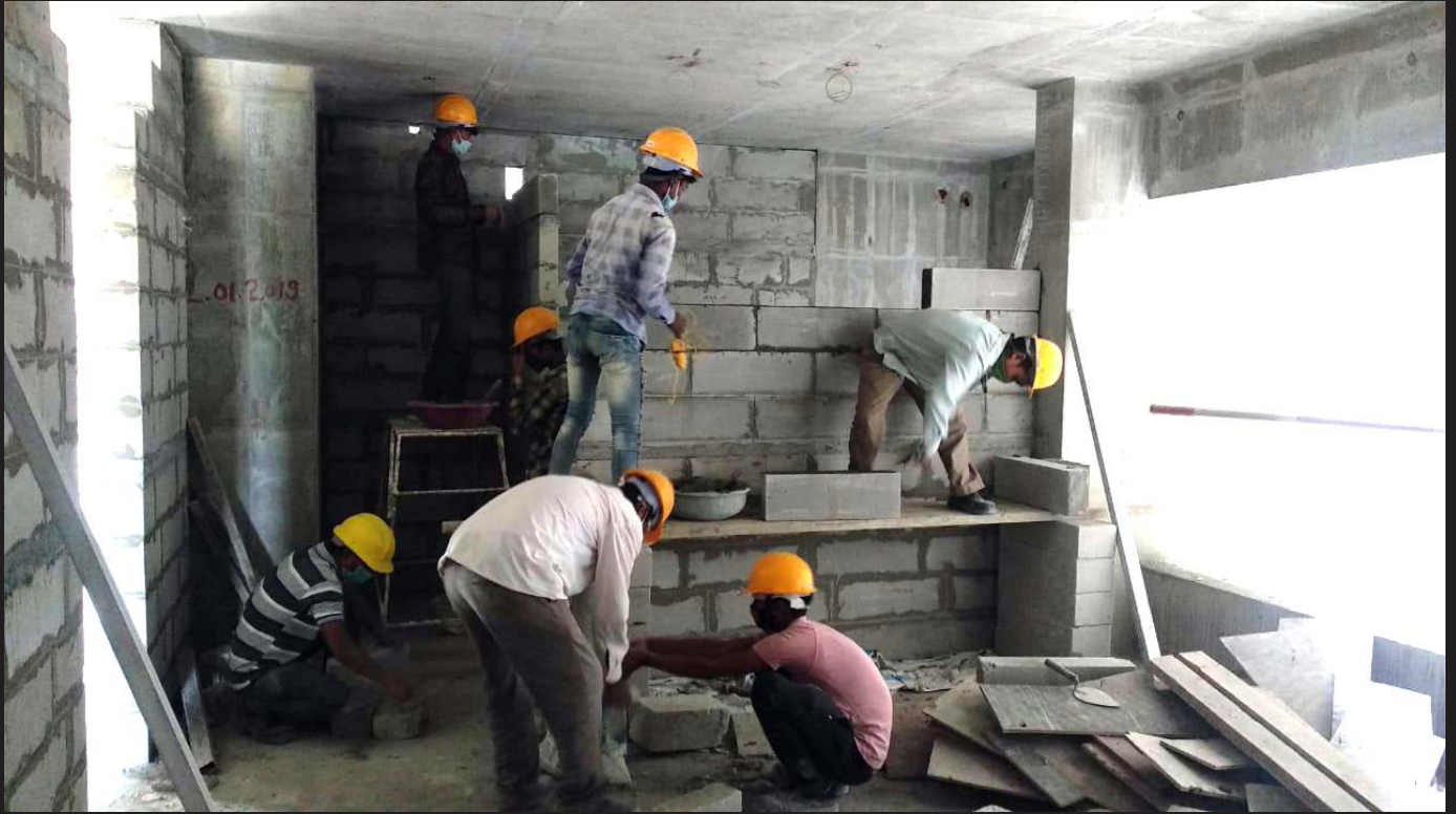
5. Block work in progress in 10 th floor
