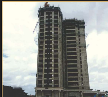
Aug 2019 - 20th floor slab
