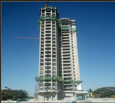
Jan 2020 - 26th floor slab
