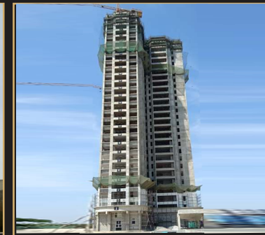
Mar 2020 - 28th floor slab
