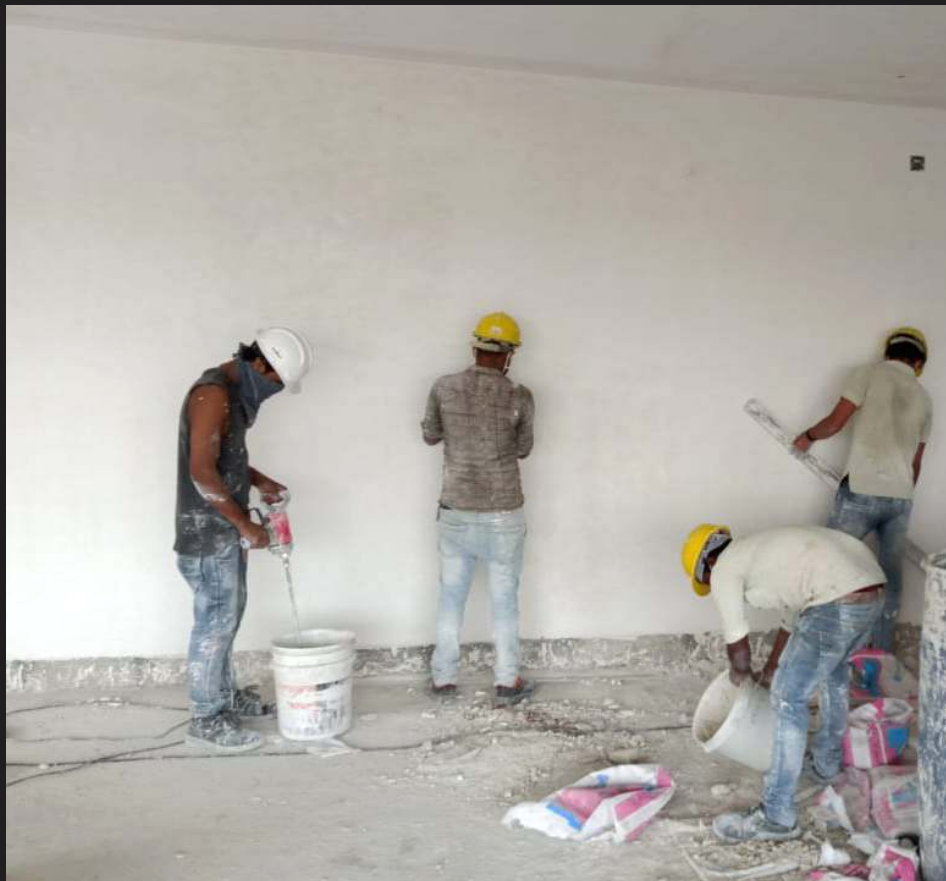
4. Internal wall plastering in 9 th floor
