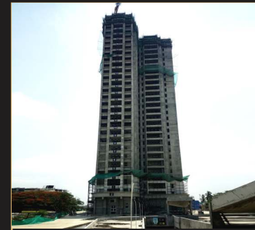
May 2020 - 29th floor slab
