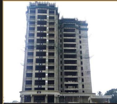
Jun 2019 - 16th floor slab
