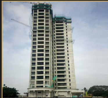
Nov 2019 - 24th floor slab
