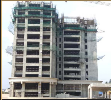
Apr 2019 - 12th floor slab
