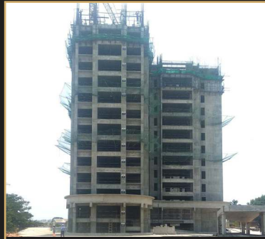
May 2019 - 13th floor slab
