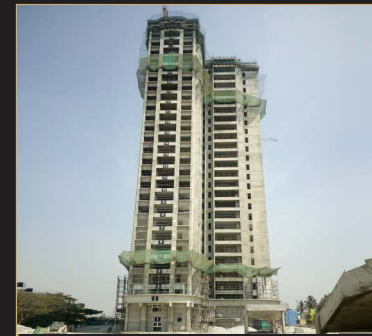
Feb 2020 - 27th floor slab
