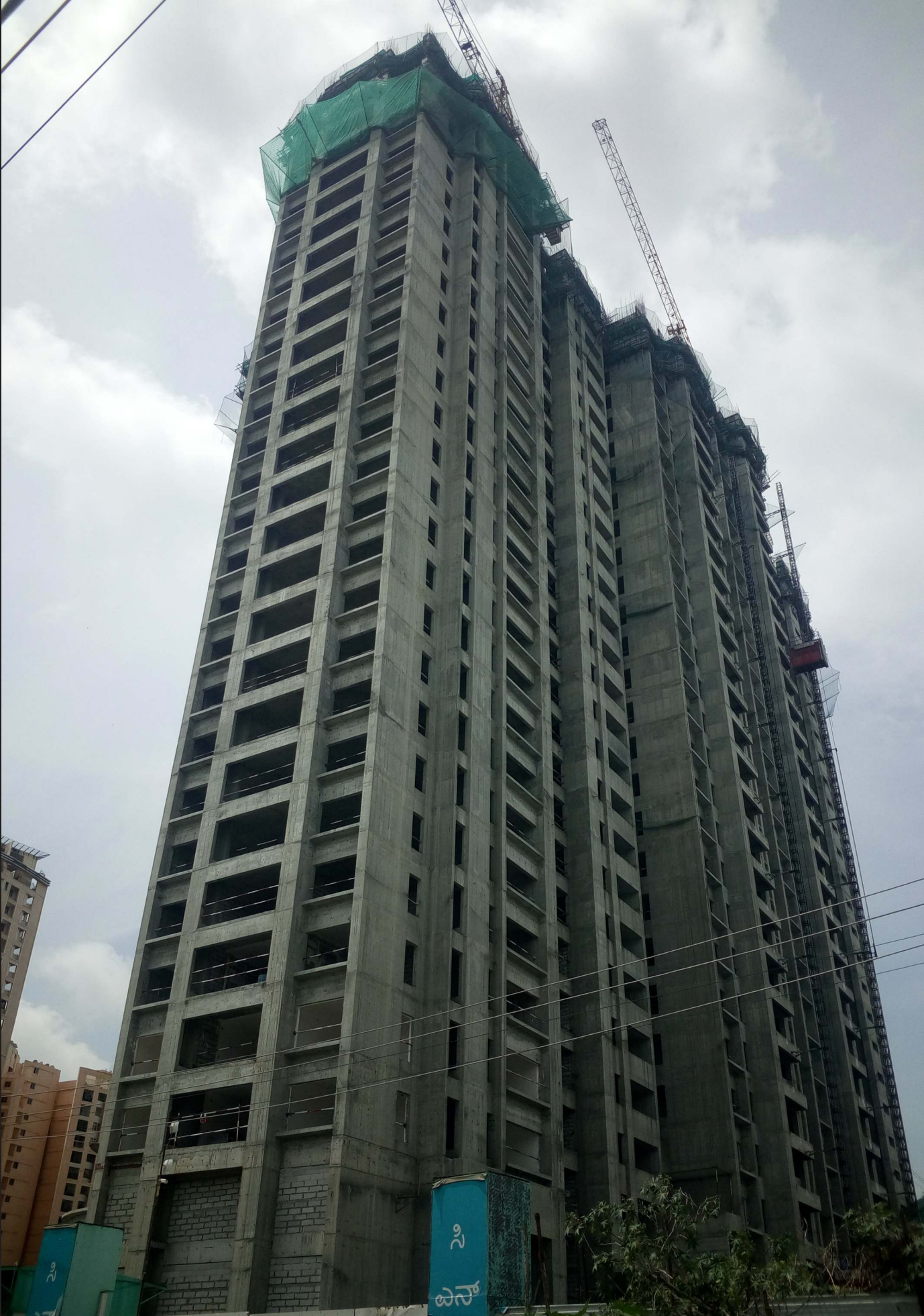
3. View from back gate
