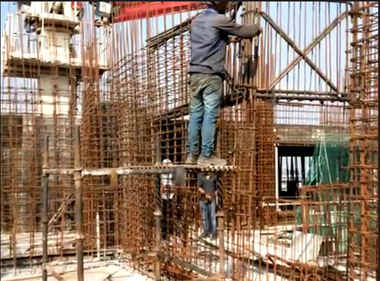
5. Rebar Structure work in progress on 30th floor Tower B
