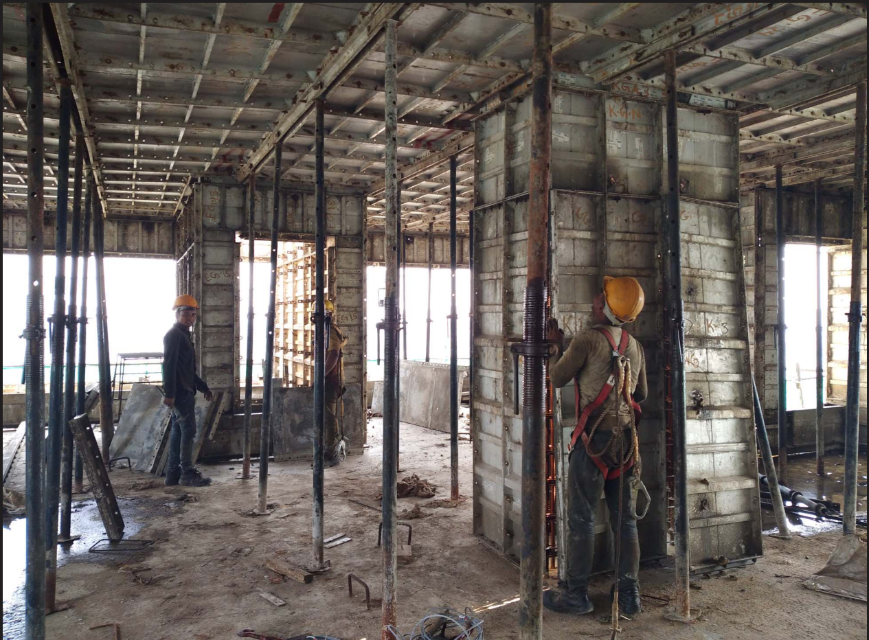
3. Deshuttinger work is in progress. on 31st floor Tower A
