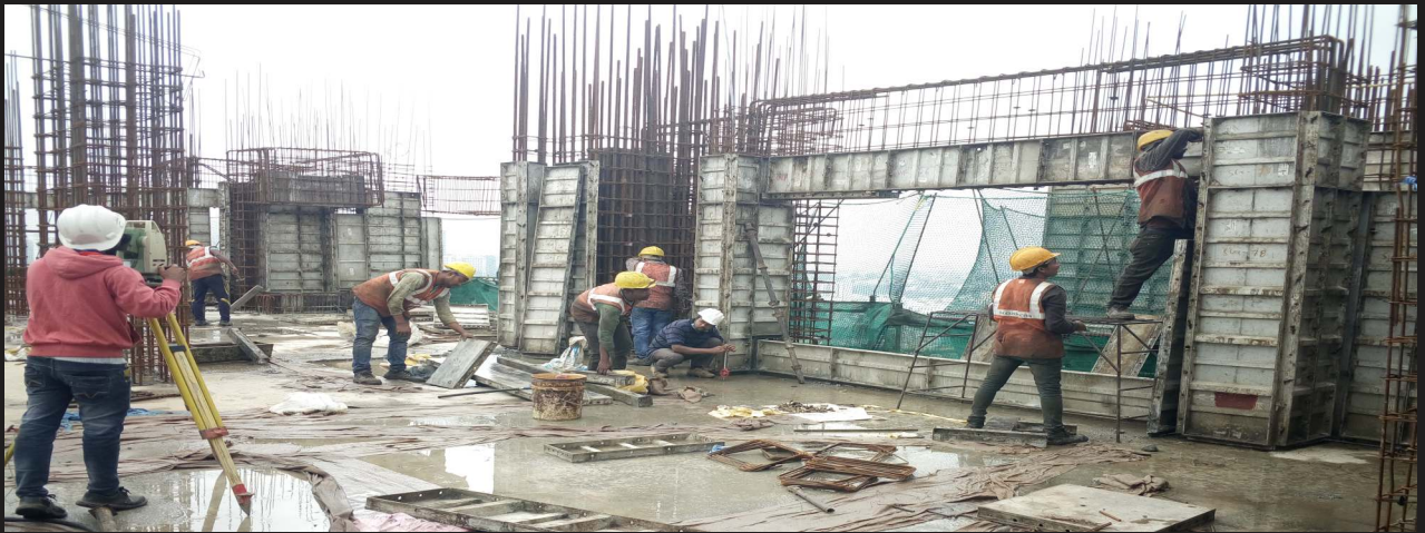
8. Shuttering work is in progress on 32nd floor Tower A
