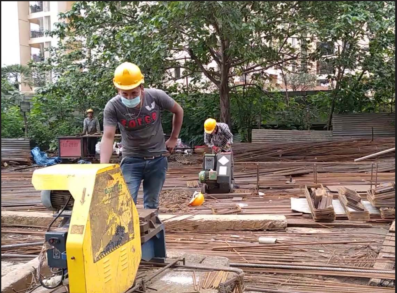
11. Bar bending & cutting in progress
