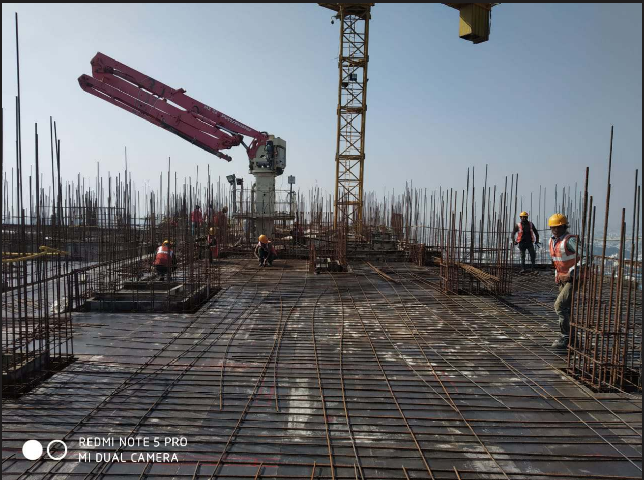
7. A-3, 32nd floor slab reinforcement work in progress
