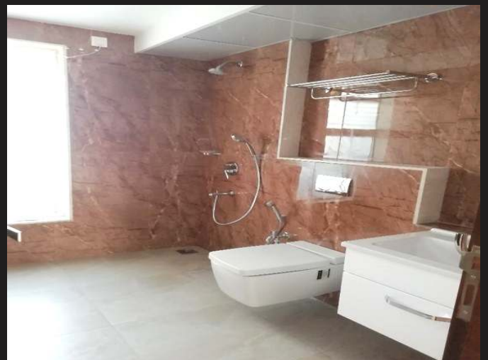
CP & Sanitary fixtures fixing work Completed
