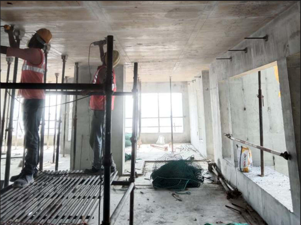
9. 32nd floor Grinding work in ceiling Tower A
