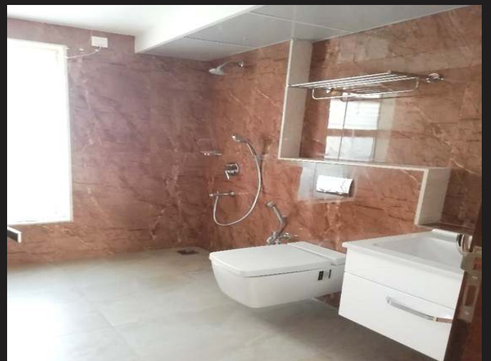
CP & Sanitary fixtures fixing work Completed
