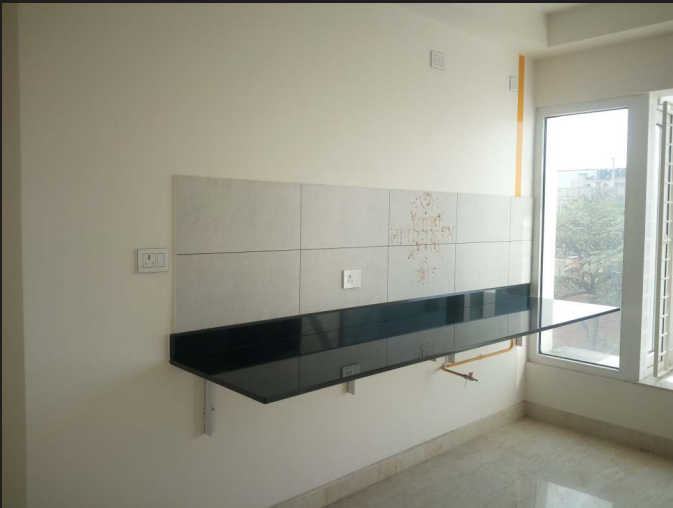
Kitchen counter slab fixing work completed
