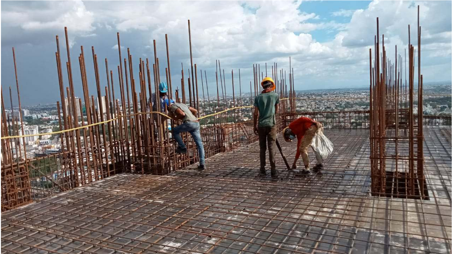
■ SLAB WORK REINFORCEMENT
