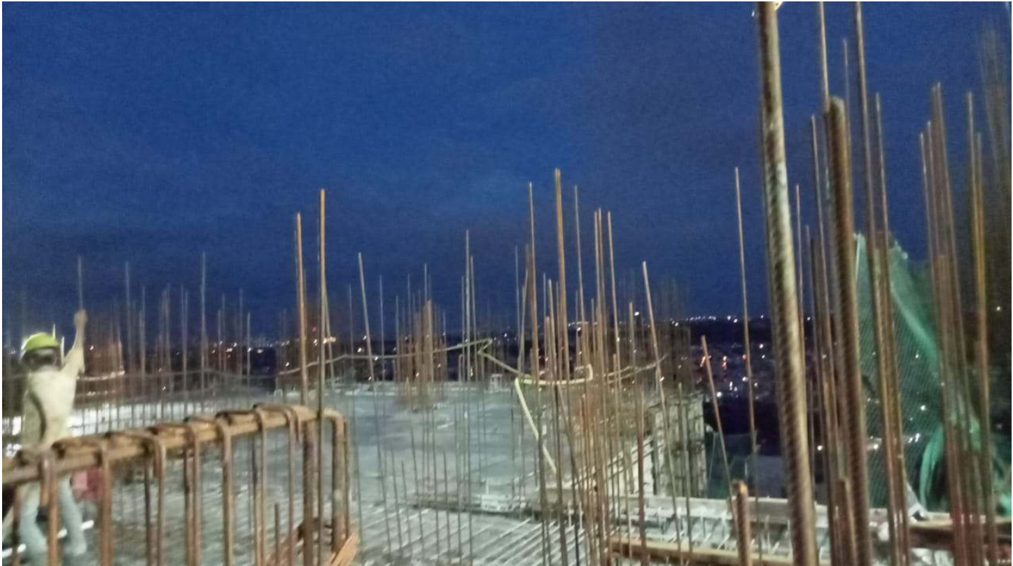
■ SLAB WORK COMPLETED
