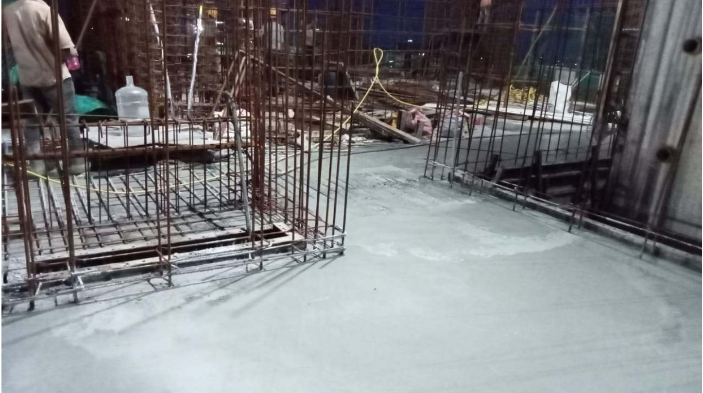
■ SLAB WORK COMPLETED
