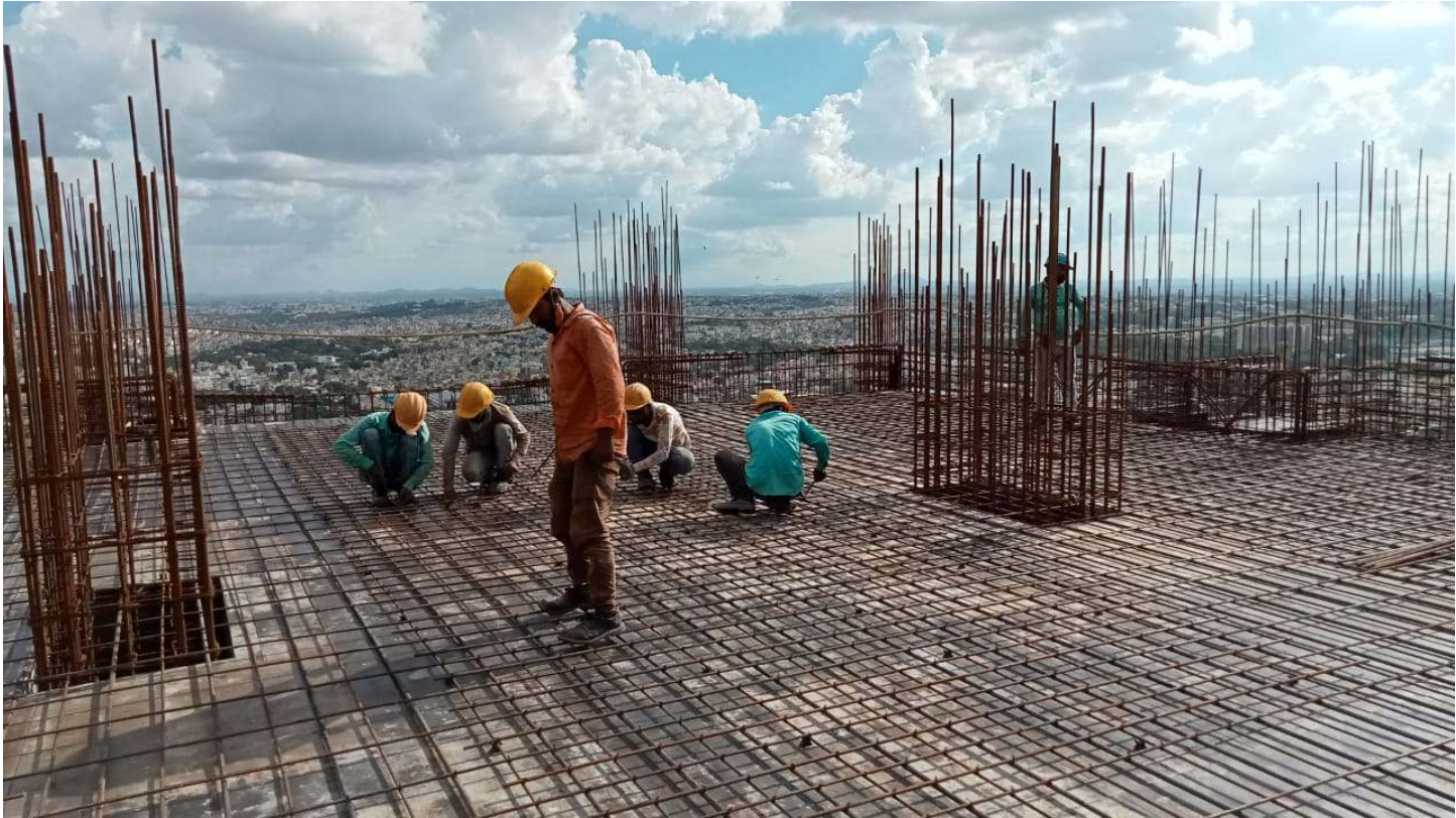
■ SLAB WORK REINFORCEMENT
