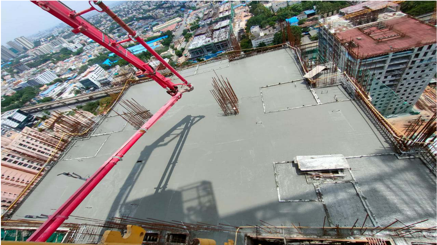
■ SLAB WORK COMPLETED
