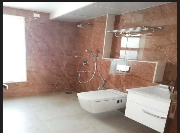
CP & Sanitary fixtures fixing work Completed
