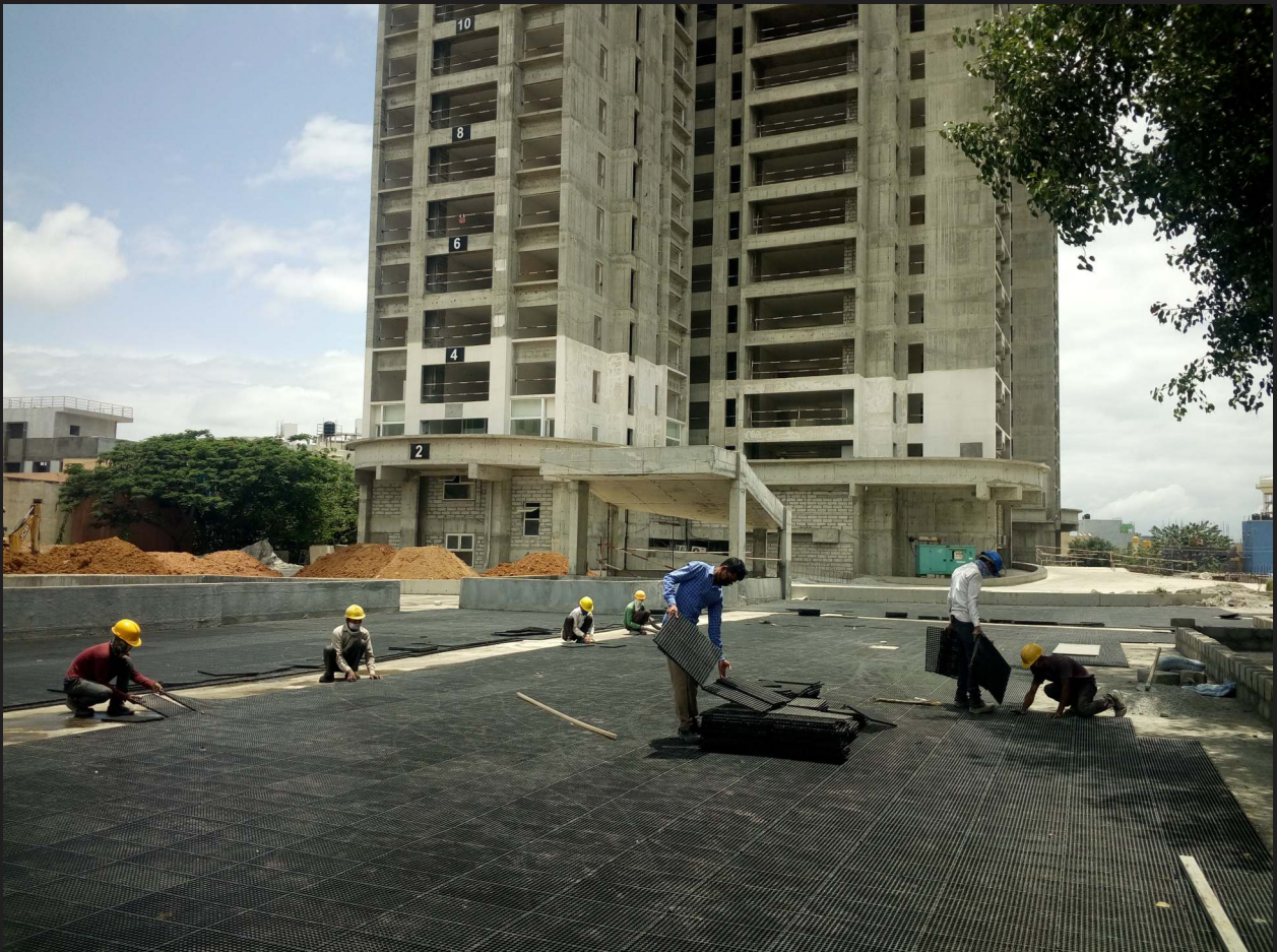
14. lawn work is progress - laying drain cell
