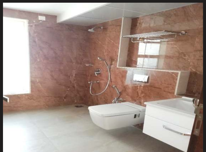
CP & Sanitary fixtures fixing work Completed
