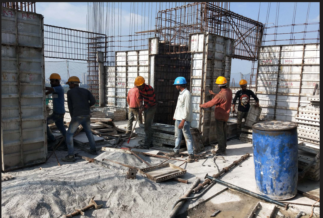
11. 40th floor shuttering work progress on Tower A
