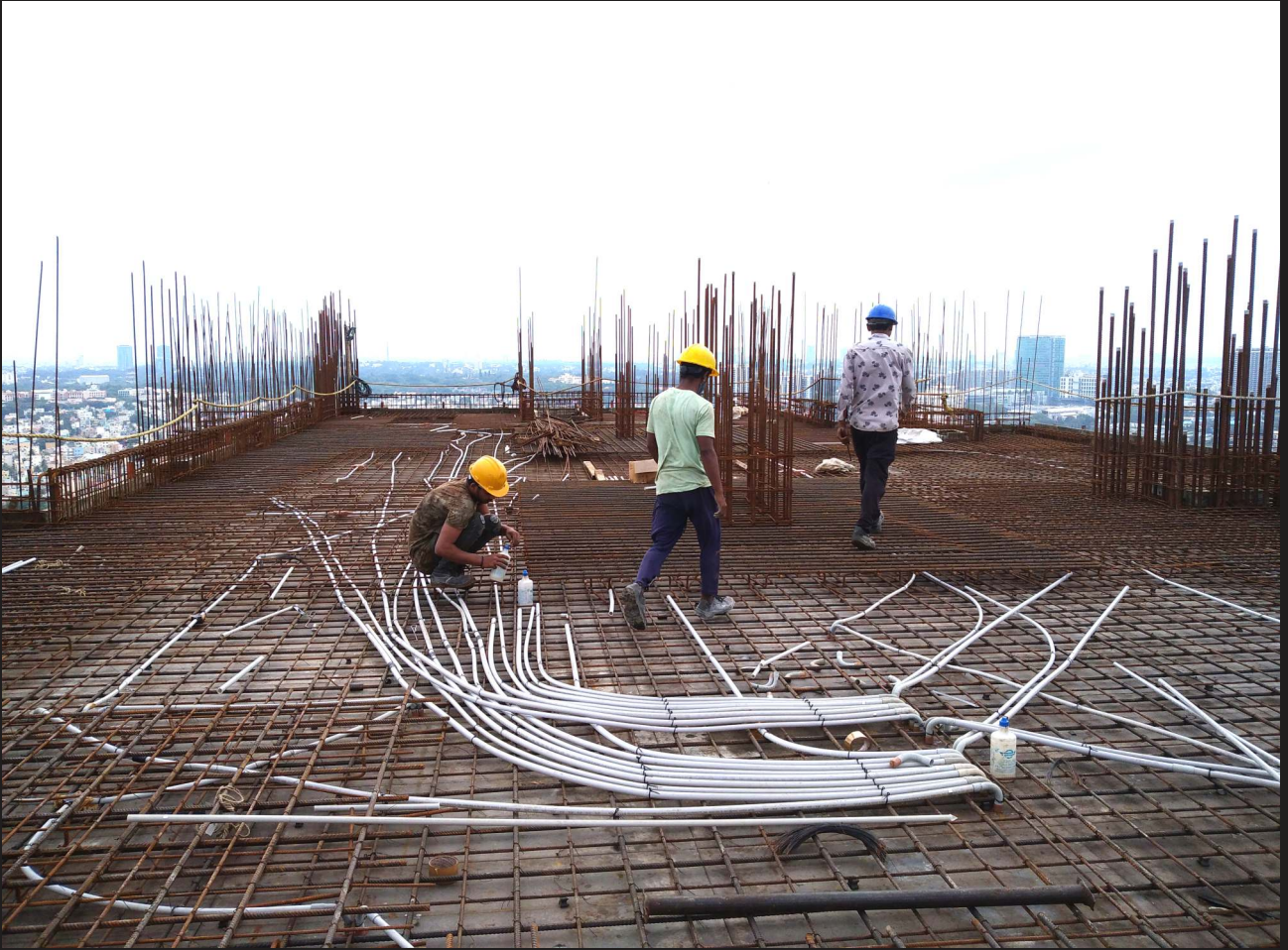
8. 39th floor shuttering work progress on Tower A
