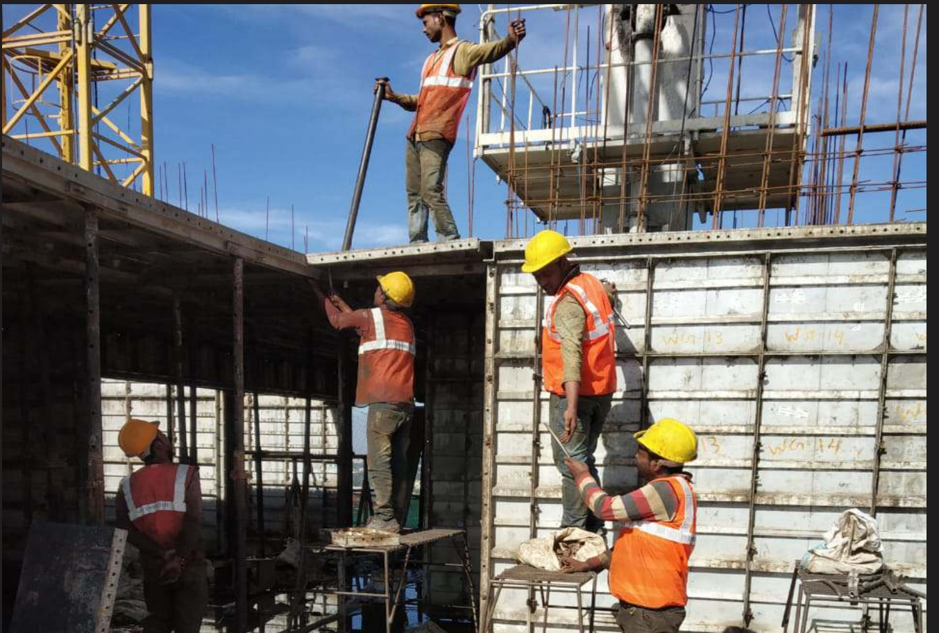
11. 36th floor shuttering work progress on Tower B
