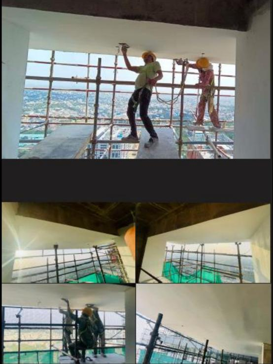
TOWER A – 45<sup>TH</sup> FLOOR PROJECTION SLAB BOTTOM POP WORK IN PROGRESS
